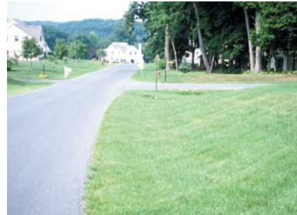
Use vegetated swales and filter strips for quantity and quality control.
