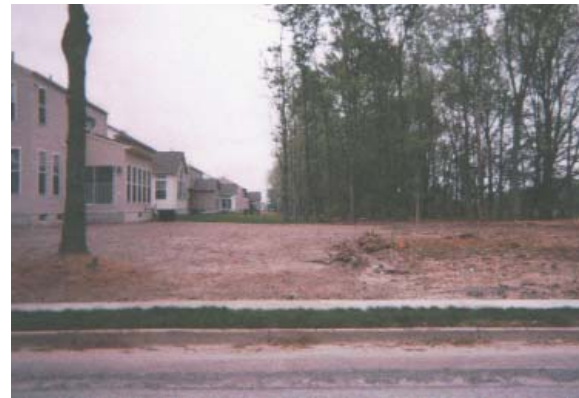
Excessive land disturbance
