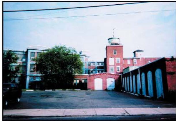
Wheaton Cotton Mill - ideal for creating mixed-use facility anchoring historic district; ripe for positive, creative development (5 photos)
