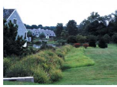
Use vegetated swales and filter strips for quantity and quality control.
