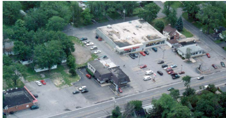
Before: Roadside Strip; parking dominates view; no shared parking; no walking environment
