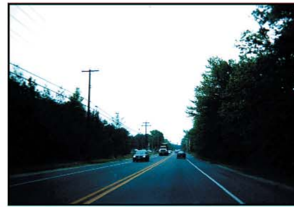
Cologne Avenue traffic signal - the signal that was supposed to solve a problem, and then created a traffic nightmare (Note: DOT plans to address underway)
