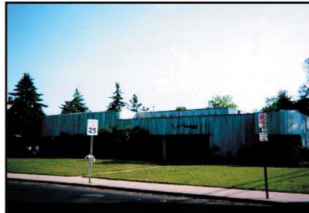
Verizon, Main Street - Inappropriate architecture for historic district (4 photos)
