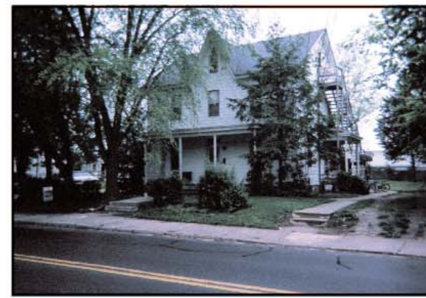
Triplex - ordinance should be created to protect old, single-family homes
