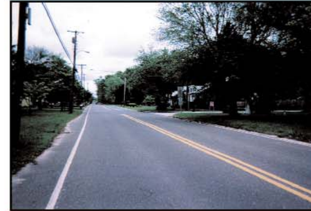
Pump Branch Road - no sidewalks
