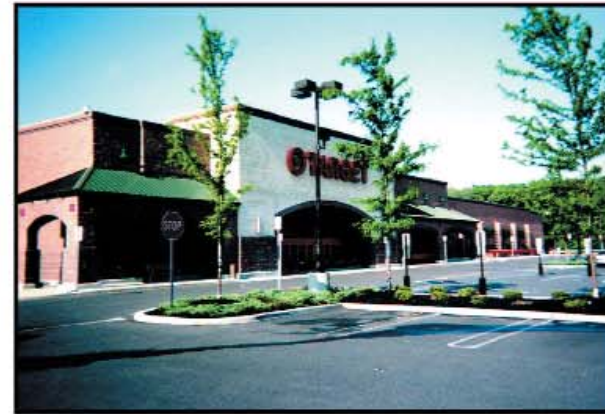
Route 73 South, Evesham Township - a not-so-boxy "big box" store
