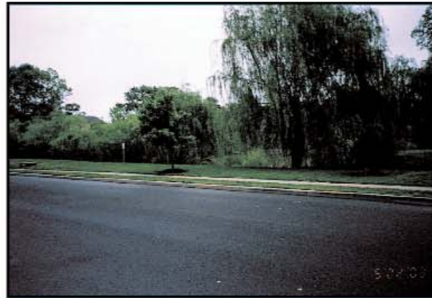
Wilton's Corner retention basin
