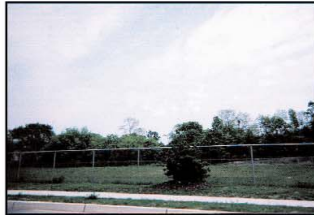
Fenced, poorly-screened basin
