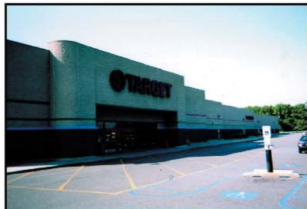
White Horse Road, Voorhees - a "big box" store designed without special architectural consideration
