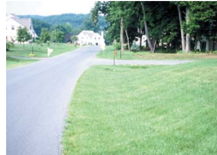
Use vegetated swales and filter strips for quantity and quality control.
