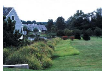
Use vegetated swales and filter strips for quantity and quality control.
