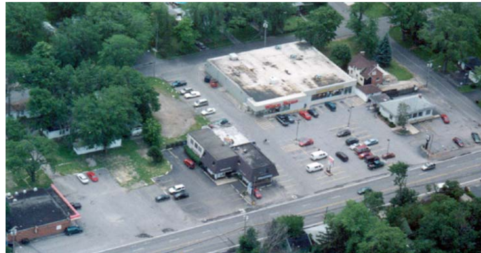
Before: Roadside Strip; parking dominates view; no shared parking; no walking environment
