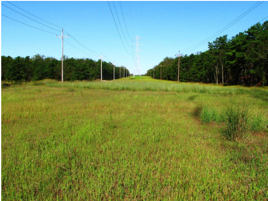
Figure 5.6. Example of a span dominated by herbaceous vegetation. The span is a food plot on a New Jersey Department of Environmental Protection, Division of Fish and Wildlife, Wildlife Management Area. The vegetation-management prescription is to mow.
