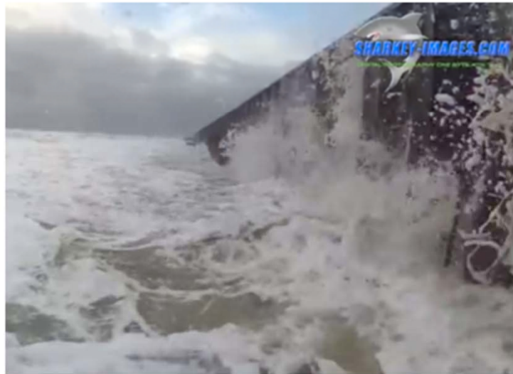
Waves crash into a sheet pile wall in Brick (Ocean County) on October 5. (Photo by Sharkey-Images).
