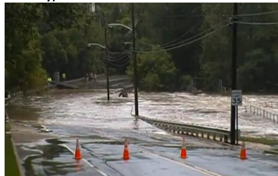
FIGURE 1 View of Inundated Pipe Bridge (to right of roadway)
