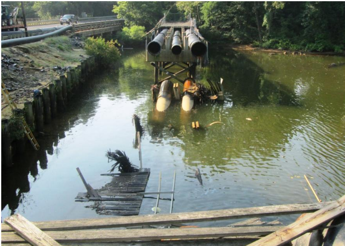
Collapsed portion of Swimming River Pipeline Bridge – View looking South. Note Swimming River Road Bridge over Swimming River and also emergency bypass lines installed on bridge and shoulder of Swimming River Road.
