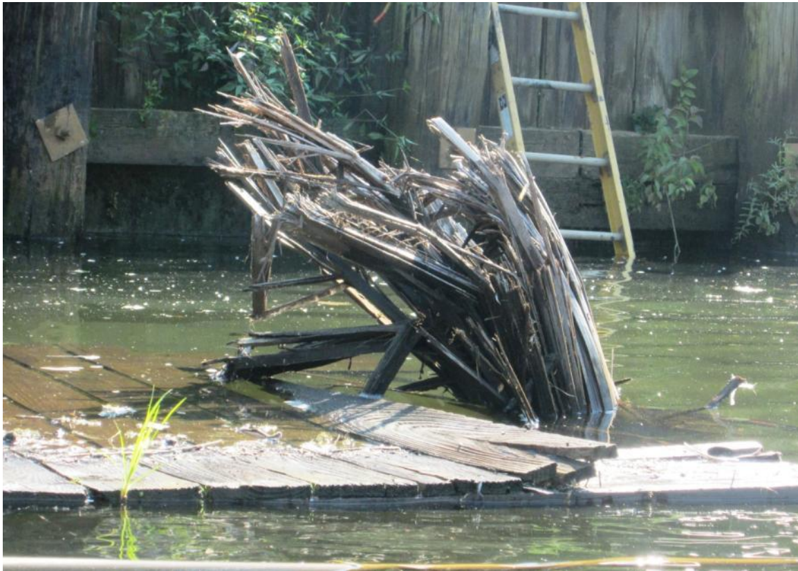
Timber Pile 5A East - Typical failed pile
