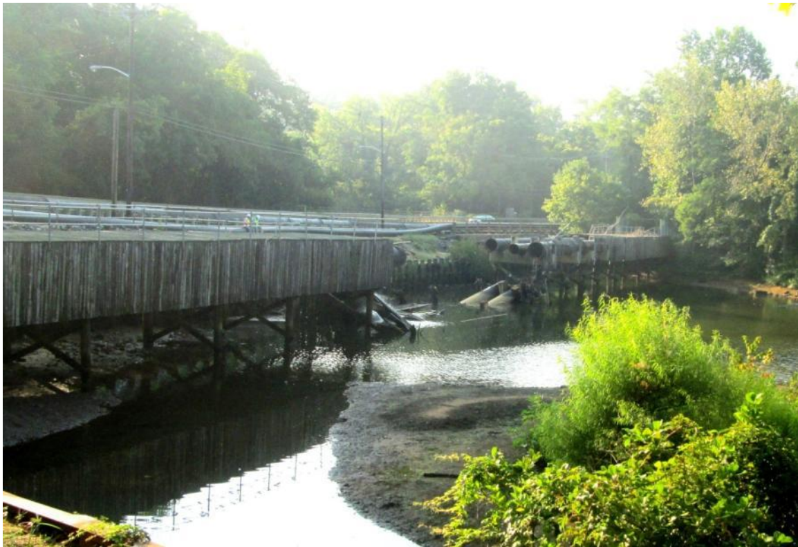
Swimming River Pipeline Bridge – August 2012. Note collapsed central portion
