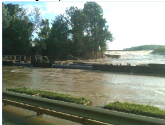
FIGURE 2 View of Inundated Pipe Bridge (beyond grassed area in the foreground)
