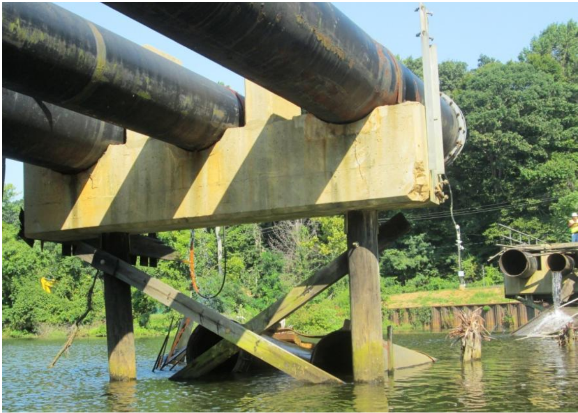
Pile Cap 6B - Typical pile bent with concrete pile cap. Note concrete cross bracing on timber piles and vertical steel channel on edge of pile cap
