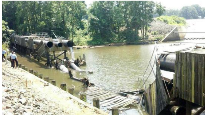
Failed Pipe Bridge
