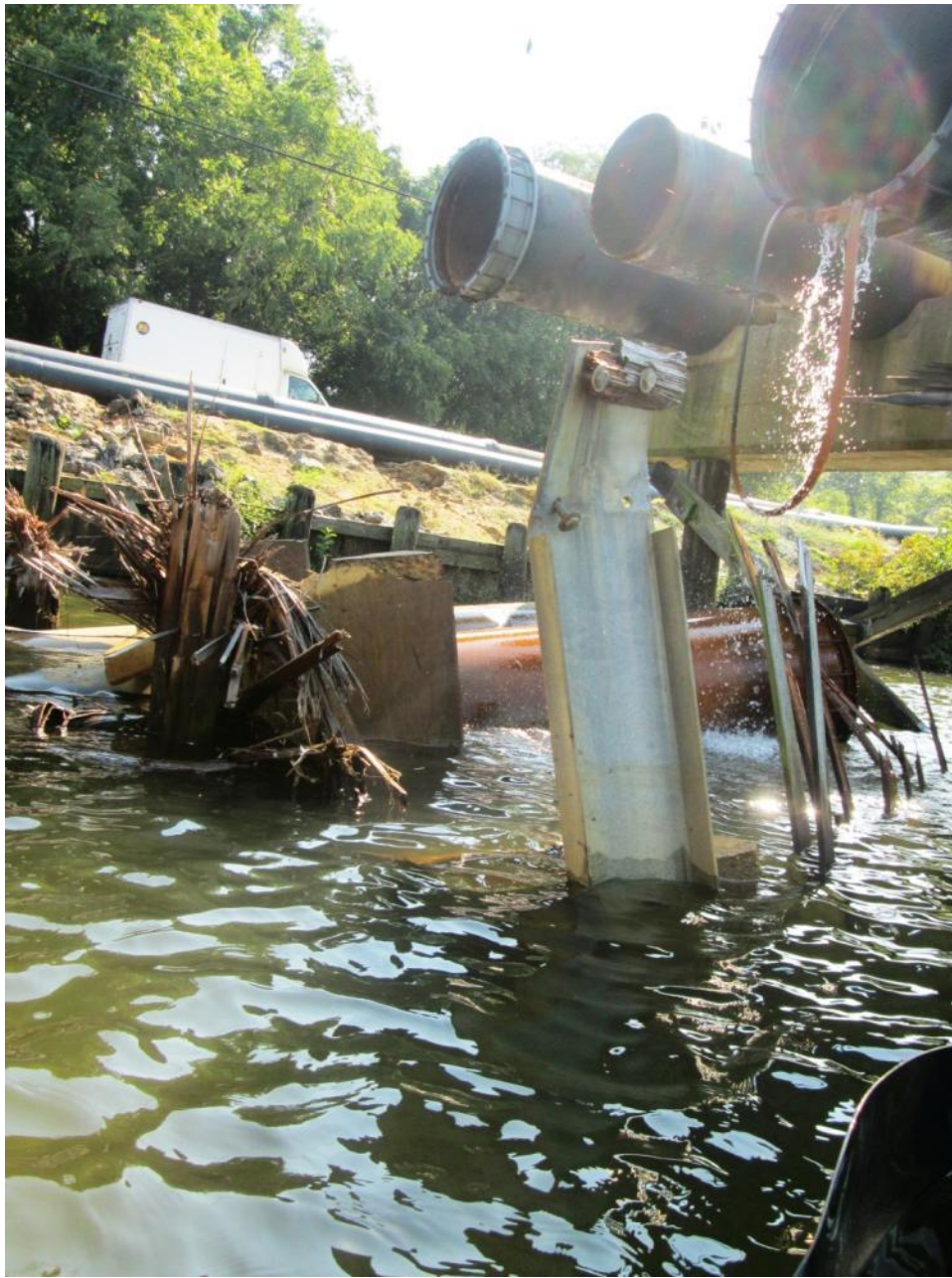
Failed Piles 6A East and 6A West (Foreground). Remaining Pile Bent 6B (Background). Steel channel used to mount timber siding seen in foreground. Channel is still attached to submerged concrete pile cap.
