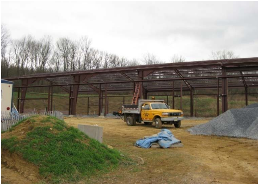
Figure 2: Progress on garage being erected using prefabricated steel.
