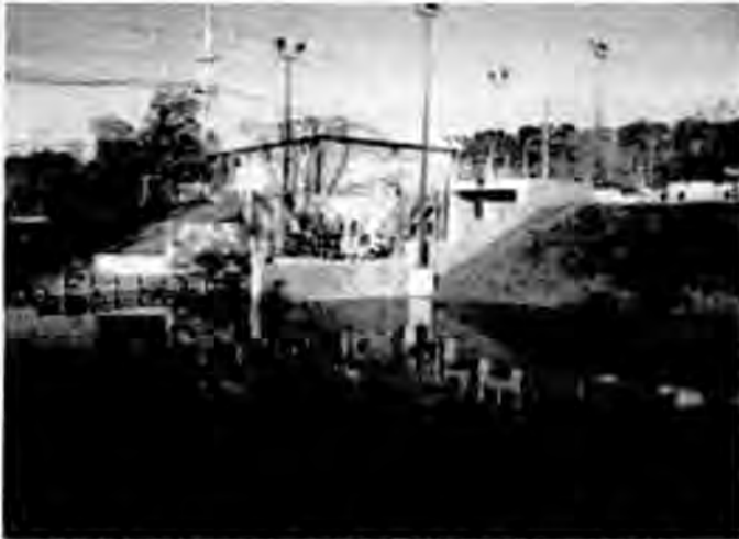
Exhibit 3.14 - 100 cfs Storm Water Pump Station Middlesex, NJ, Designed by AECOM(URS)
