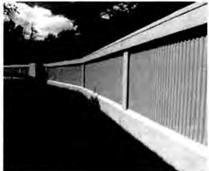
Exhibit 3.11 - Flood Wall Middlesex, NJ - Designed by AECOM(URS)
