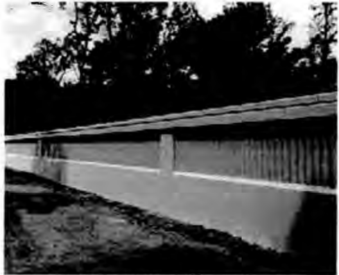
URS Designed 1900 LF of Composite Sheet Pile and Tee Floodwall, Middlesex Borough NJ
