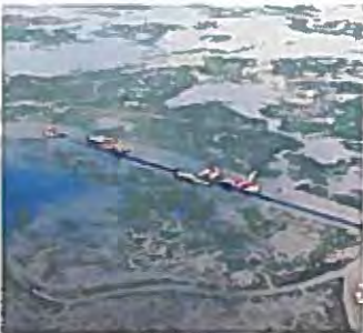
Building a barrier to protect New Orleans from future storms
