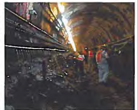
MTA Capital Construction Montague Tunnel Restoration
