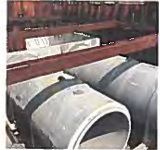
We provided construction oversight at the USACE-New York District's Sandy Hook to Barnegat Bay Beach Erosion Control project, including dewatered construction of twin 8-foot RCP outfall extensions.
