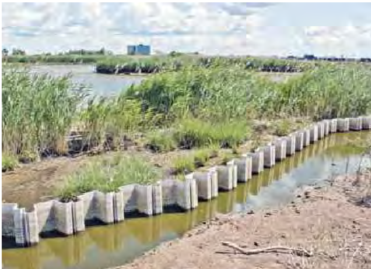
5 Concept Image of Proposed Vinyl Sheet Pile Armoring
