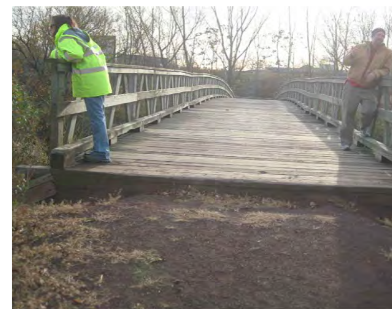
2 Existing Pedestrian Bridge: Fill and stabilize access point per trail detail. Smoothly grade trail to meet bridge El. 6.5
