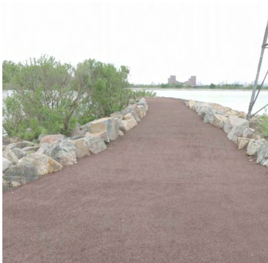
2 Concept Image of Proposed Stone Curb & Rip-Rap Armoring
