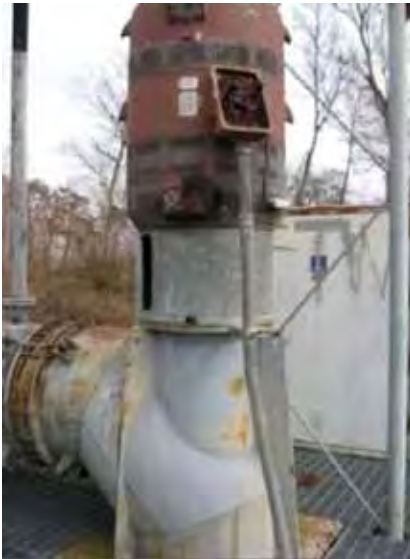
CDM Smith’s activities included selected site inspections of damaged facilities in an effort to prioritize projects.
