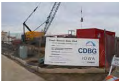
Downtown Des Moines was served by a combined storm and sanitary sewer system resulting in localized flooding during heavy rain events, especially during high river levels. The CDBG-DR funded project constructed a separate storm sewer system and storm water pump station to serve this area.
