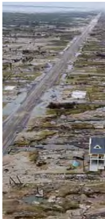
Highway 87 on the Bolivar Peninsula sustained heavy damage in Hurricane Ike. CDM Smith is helping to coordinate funding sources needed to restore and elevate this critical roadway.
