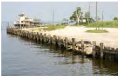
The Madisonville Bulkhead Project in St. Tammany Parish, Louisiana is being constructed using CDBG funds managed by CDM Smith.
