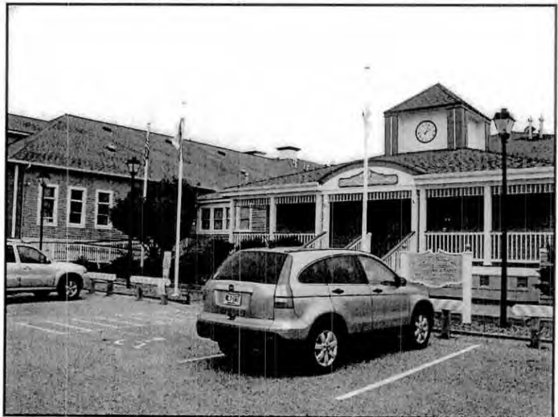
The existing Municipal Building (pre-construction).
