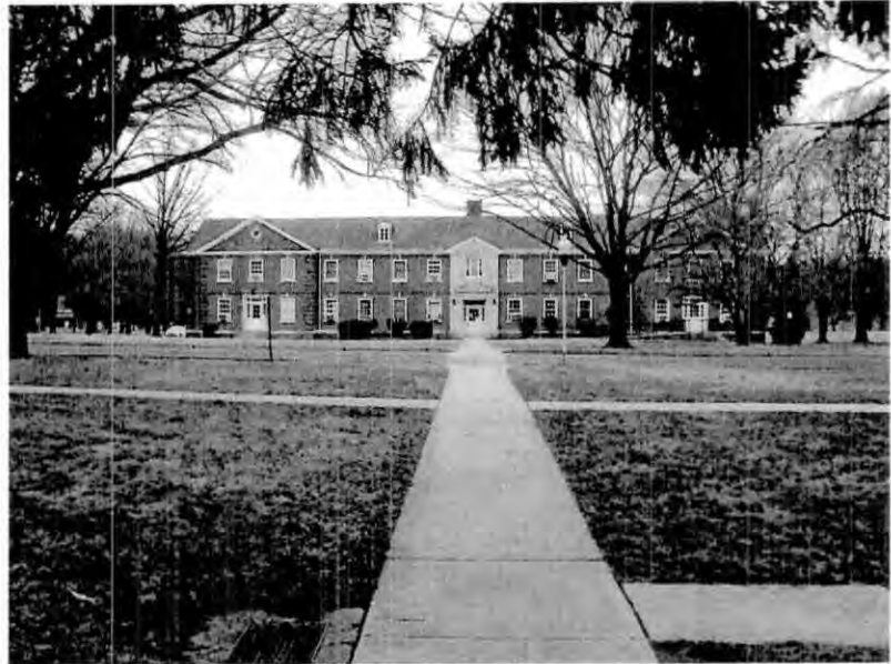
Existing Katzenbach Campus Lighting
