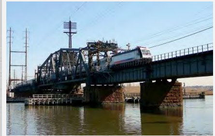
► NEC Capacity Improvements Portal Bridge Replacement, NJ
