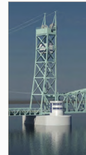
SUPPORT ON TOWERS
