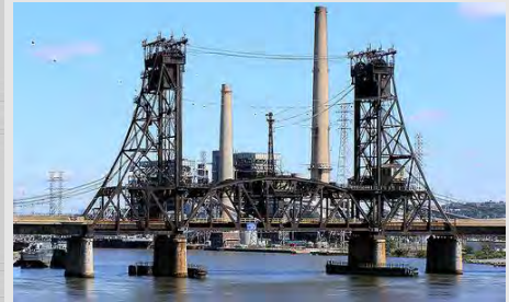
Lower Hack Lift – Built in 1928 NJT Morristown, Gladstone & NJ
