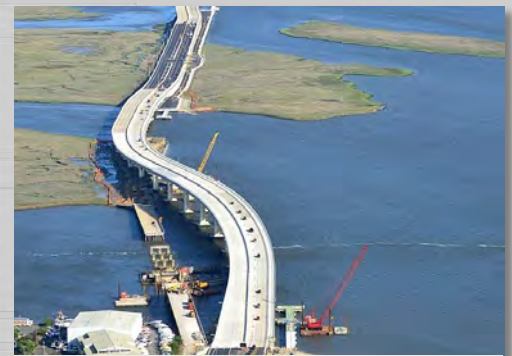
Mr. Mankbadi led foundation design for Route 52 Causeway
