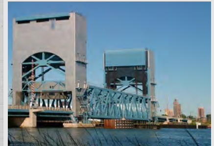
Tomlinson Bridge (2002) Highway and Freight Rail
