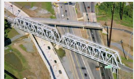
► Minimizing Public Impact NSR Bridge Replacement, PA
