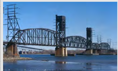
Delair Vertical Lift Bridge – Built in 1960 NJT Atlantic City Line
