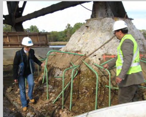
Ms. Szumanski assisted in resolving complex field problems on the Navesink River Bridge project.
