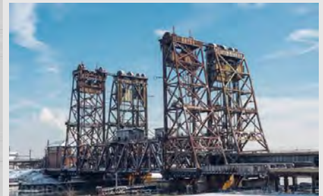
Dock Vertical Lift Bridge – Built in 1935 NJT Northeast Corridor
