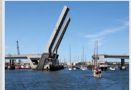
Port River Bridges, Australia (2008) Freight Rail
