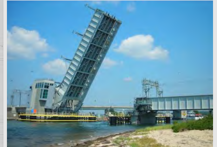
Niantic River Bridge, CT (2013) Northeast Corridor
