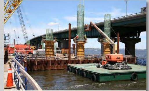
Mr. Schetelich is managing the replacement of Great Egg Harbor Bridge, currently in construction
