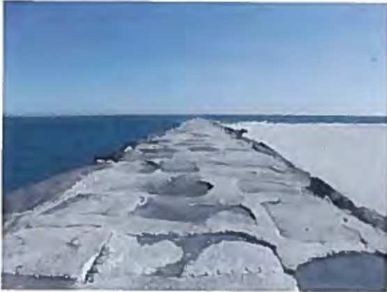
Top of Jetty Looking East
