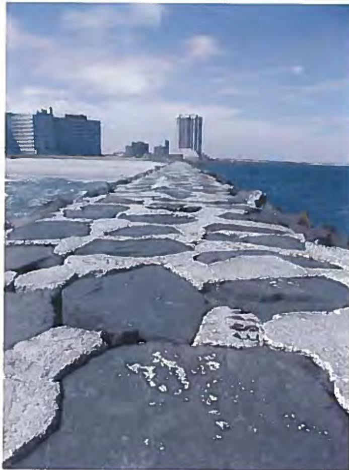
Top of Jetty Looking West
