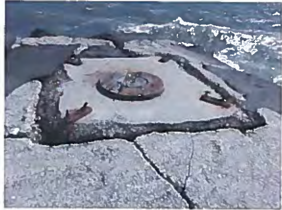
Navigational Light Tower Footing
