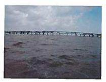
Route 37 over Barnegat Bay Hydrographic Survey; 2013; \$25K. Churchill was retained by Parsons Brinkerhoff to perform a hydrographic survey of the Route 37 over Barnegat Bay Bridge (Mathis Bridge). As a result of Hurricane Sandy, significant scour was found around six substructure units located at the east end of the structure. Churchill performed a hydrographic survey of the structure, upstream, downstream and around substructure units, prior to the installation of scour counter measures.
