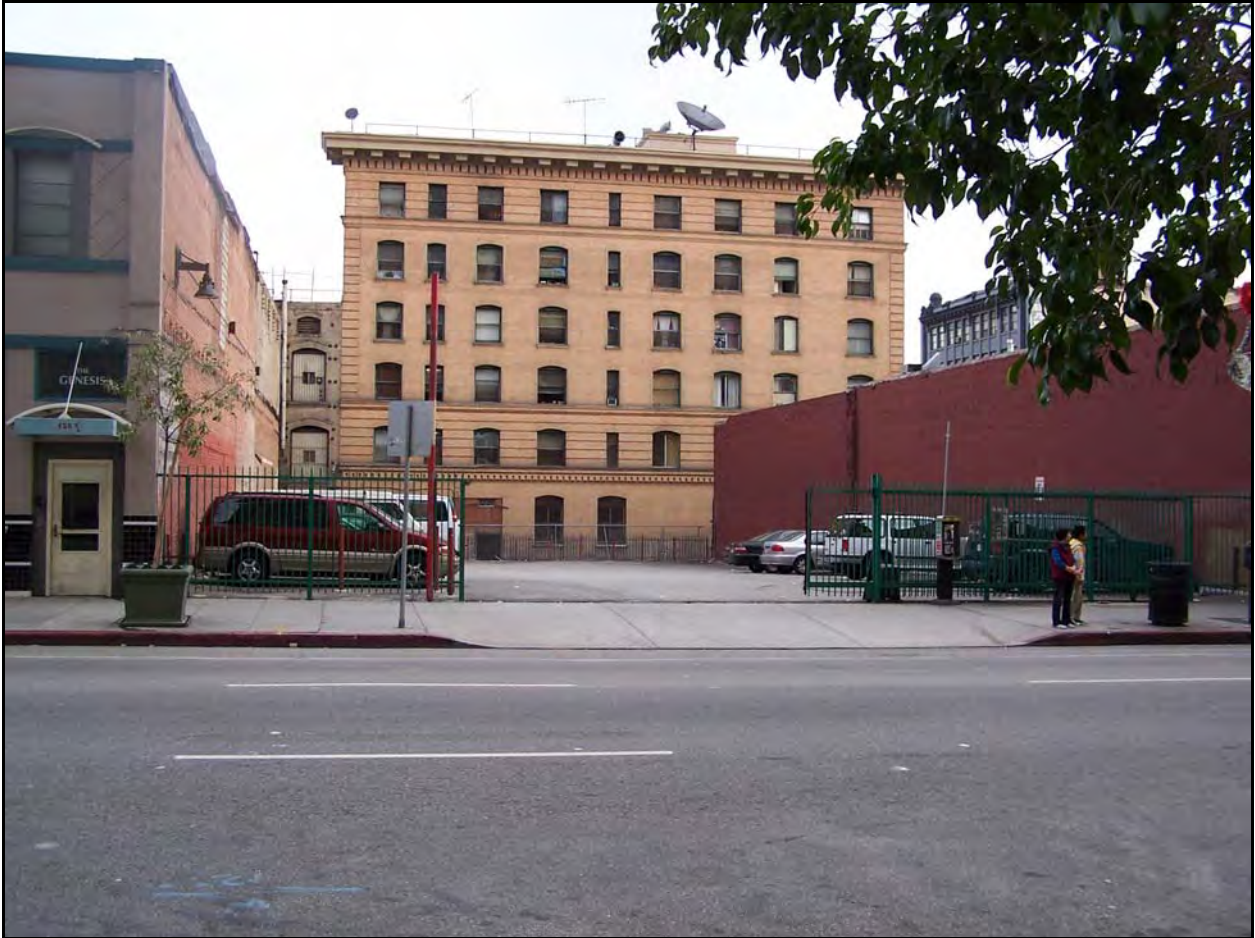
Photo 2: Existing surface parking lot with King Edward Hotel visible in the background – View southeast from west side of Main Street.
