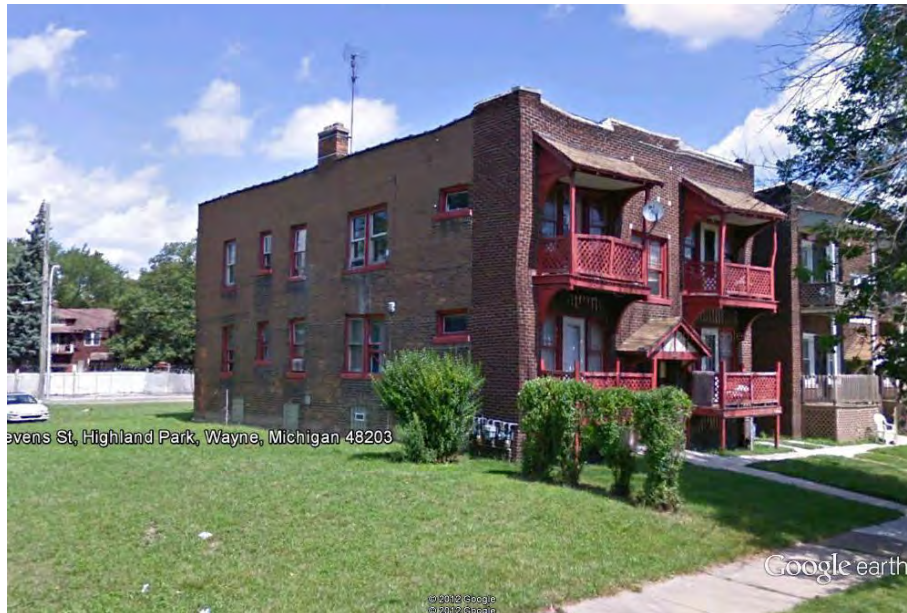
135 Stevens Street: View northeast
