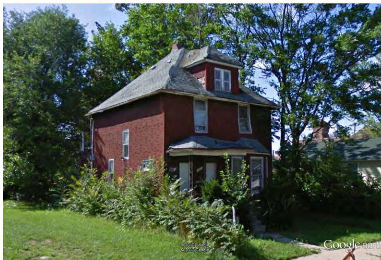
104/106 Cortland Street: View Southwest
