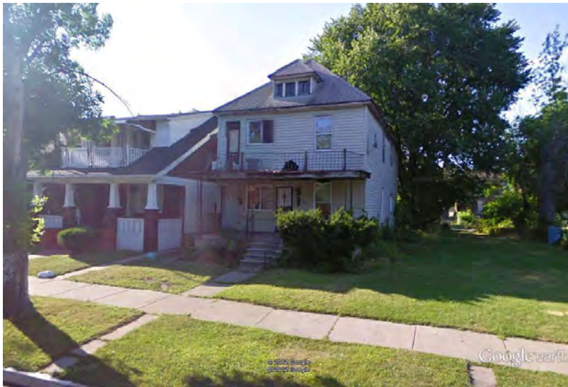
359/361 Cortland Street: Northwest Elevation
