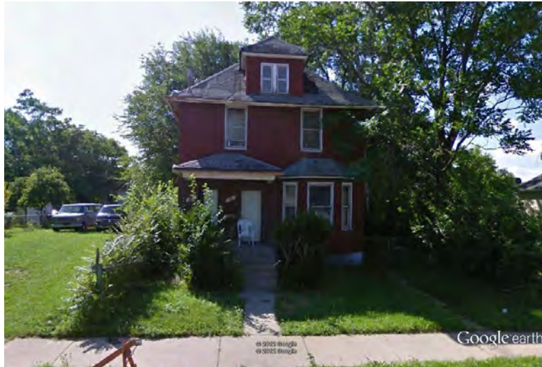
104/106 Cortland Street: Northwest Elevation
