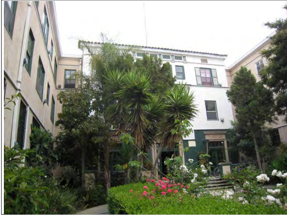
West Elevation, Looking East at Center Section
