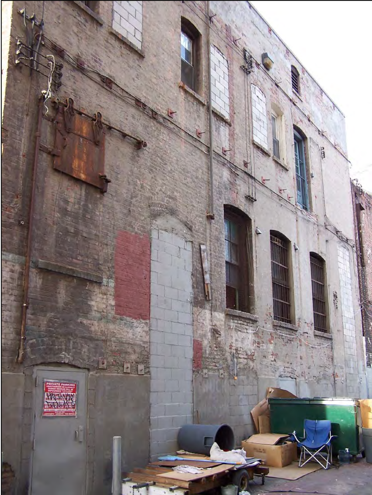
Photo 3: Back of existing Genesis Hotel building – View from Werdin Place Source: ICF Jones & Stokes, December 2009
