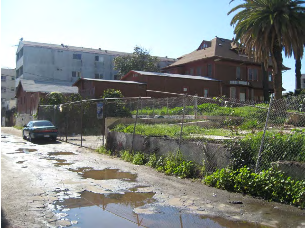
Photo 4: Rear Asphalt-Paved Area—View Southwest from Rear Alley East of the Project Site
