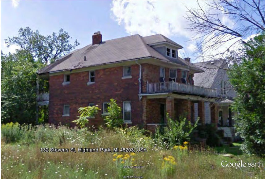
132 Stevens Street: view northeast
