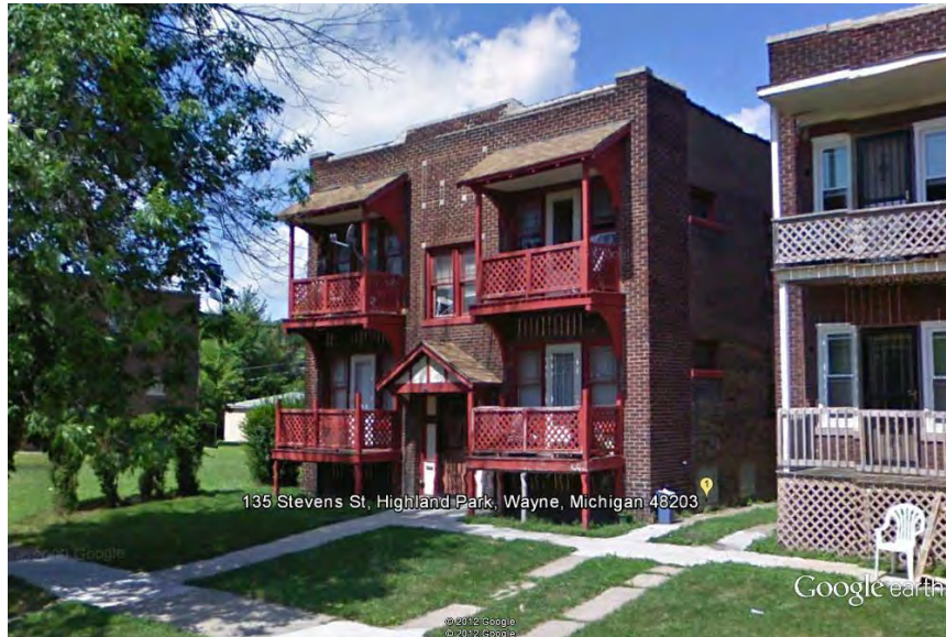
135 Stevens Street: Southeast Elevation
