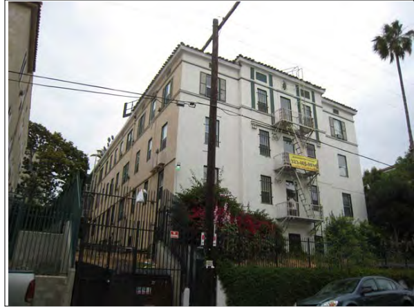
West Elevation, Looking Southeast at North Section
