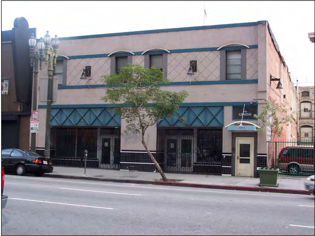
Photo 1: Existing Genesis Hotel building – View southeast from west side of Main Street
