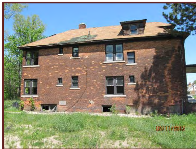
356 Elmhurst Street: view southeast
