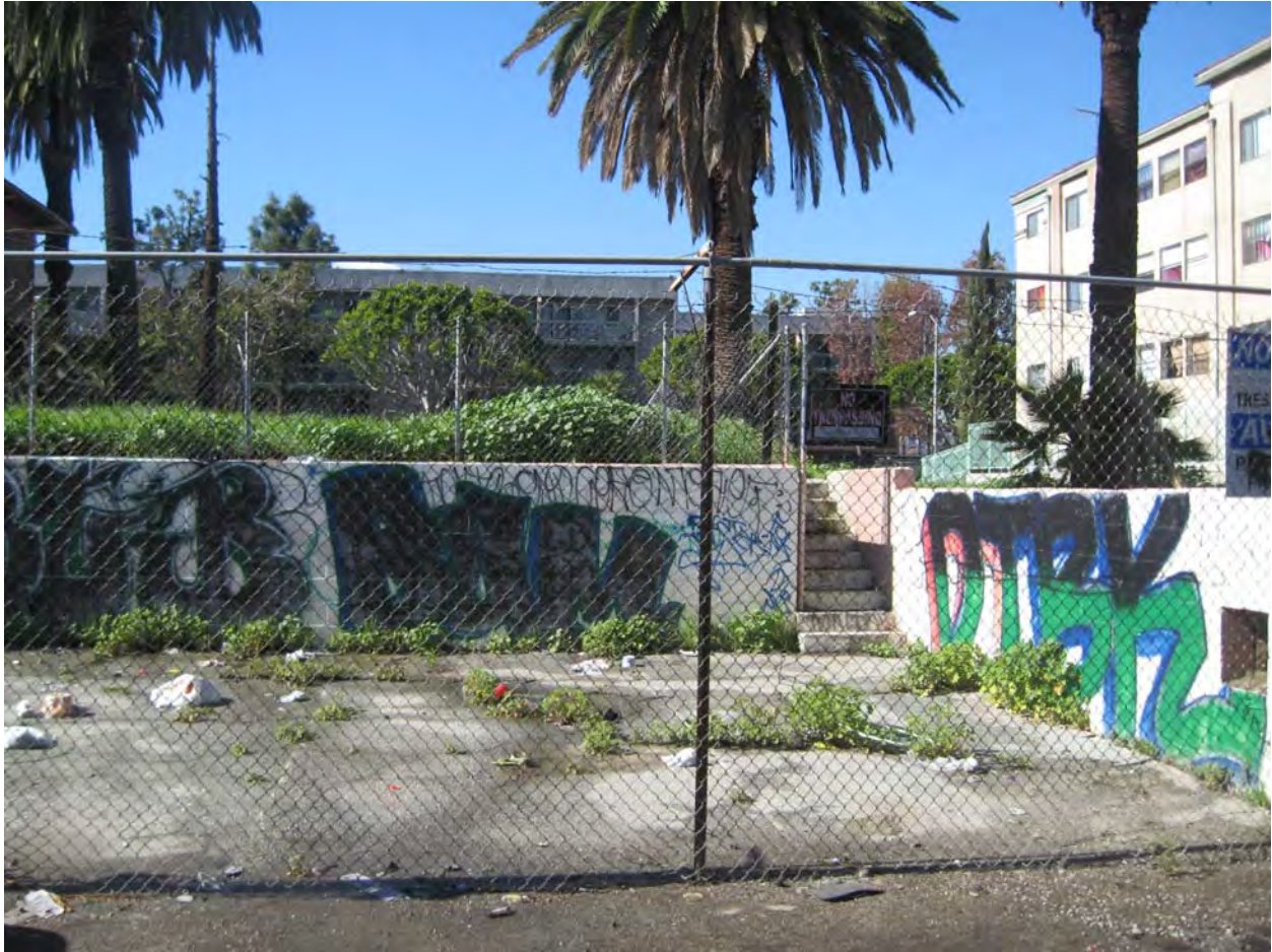
Photo 5: Asphalt-Paved Area at Street Level with Retaining Wall for Uneven Terrain— View Looking West from Rear Alley
