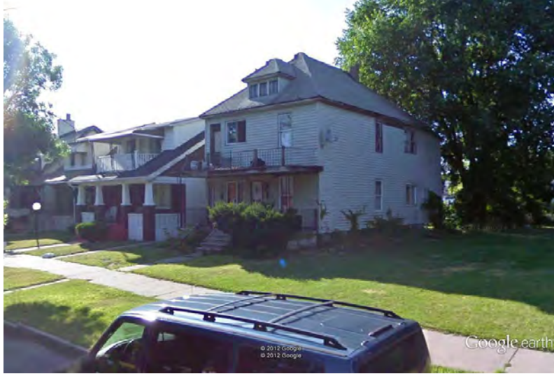
359/361 Cortland Street: view Southeast
