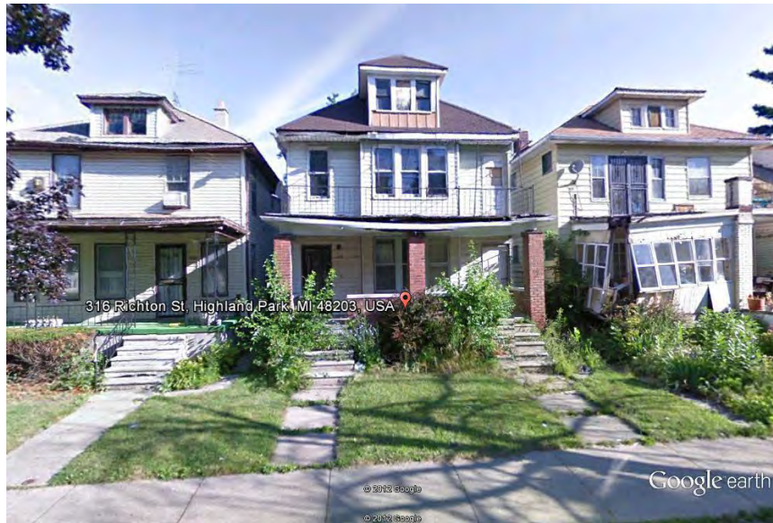
316 Richton Street: Southeast Elevation
