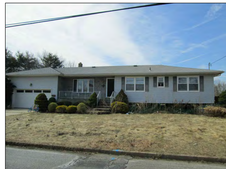
PHOTO LOOKING WEST, FRONT
