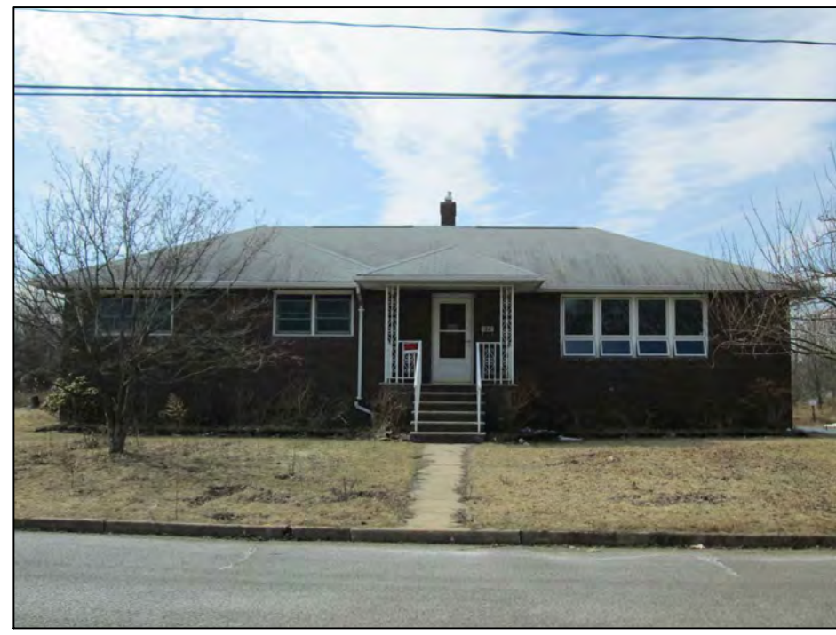
PHOTO LOOKING WEST, FRONT
