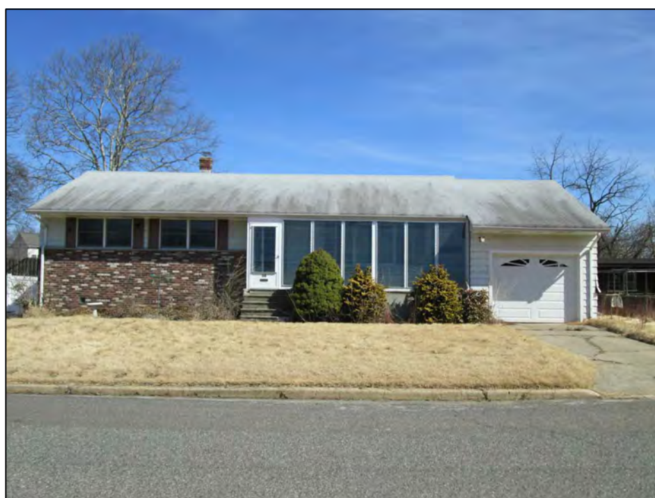
PHOTO LOOKING EAST, FRONT
