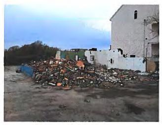
Mott MacDonald prepared the specification for the abatement/removal of these materials as well as the full demolition of the structure and all man-made site features. Mott MacDonald, on behalf of the Green Acres Program, released the specification to qualified contractors to obtain bids for the abatement of hazardous building material/ universal waste survey and the full demolition and site restoration.
