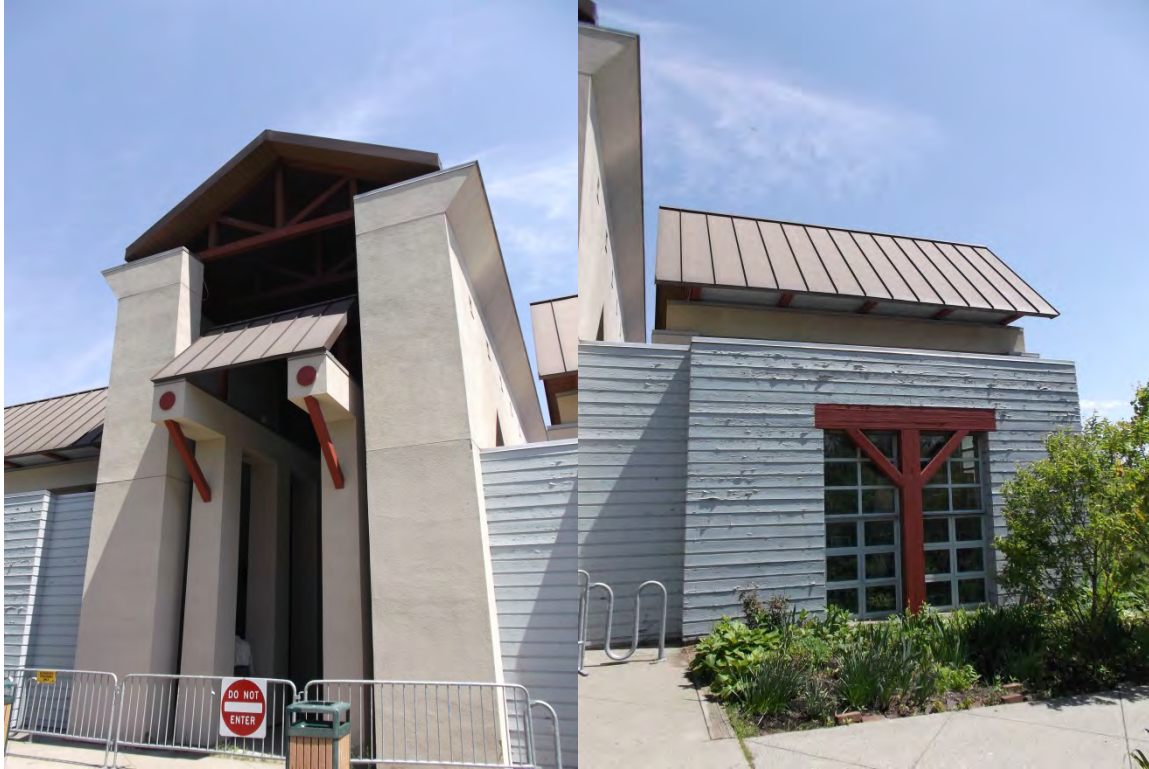
ENTRANCE AT SOUTH ELEVATION
