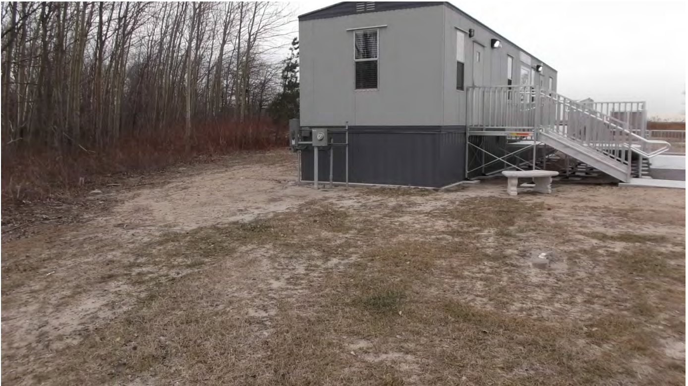
View of temporary office trailer looking west. Note finished floor height about 5 feet above ground.
