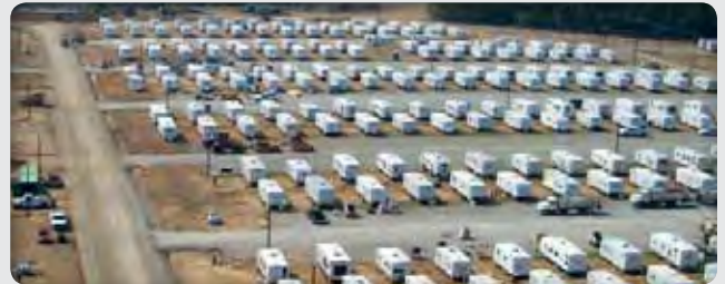
CB&I constructed a 573-unit temporary housing site at Groom Road in Baker, La., after Hurricane Katrina.
