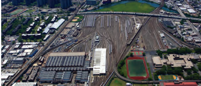
At 110 acres, Coney Island Yard is among the world's largest rail yards.
