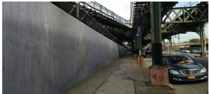
To protect the perimeter of the yard on a short-term basis, STV designed a temporary 12,000-lf wall.
