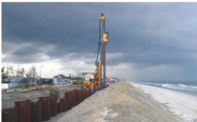
For this successfully completed sea wall project, MM provided a full range of engineering services, from emergency planning through construction.
