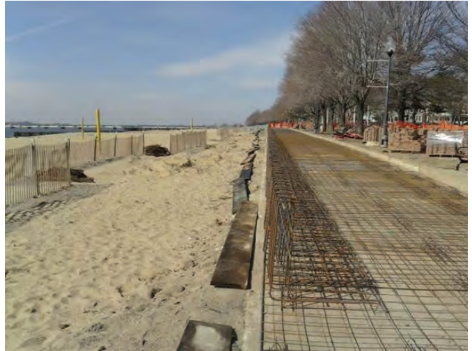
MM was extensively involved in post-Sandy reconstruction work in Perth Amboy, NJ.
