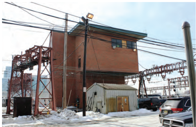
STV performed surveys and condition assessments of all structures and systems for restoration of the historic Hoboken Terminal and Yard.
