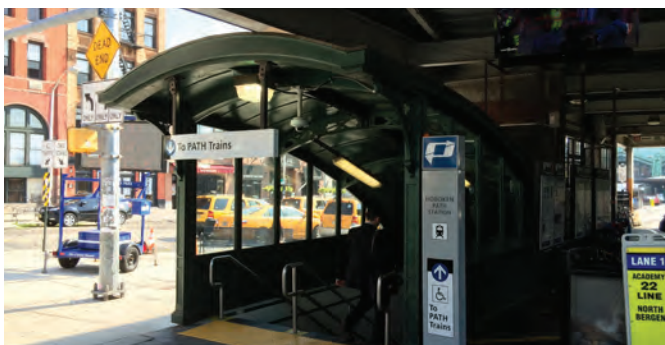
Hoboken Station: STV evaluated barrier options as part of a flood resiliency study focusing on exterior stairways.
