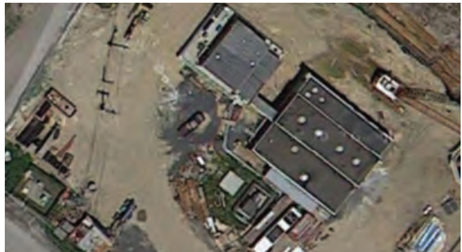
Following Hurricane Sandy, MCUA relied upon MM to restore the Edison Pump Station and protect it from future storms via a flood wall.
