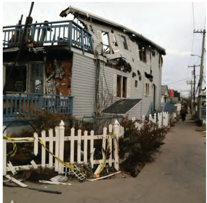
STV has extensive post-Sandy experience (NYC Department of Buildings assignment shown above).
