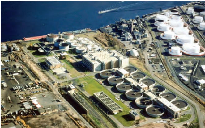
MM has extensive experience at PVSC's facilities, spanning more than 40 years, including a long list of projects in the last decade alone.
