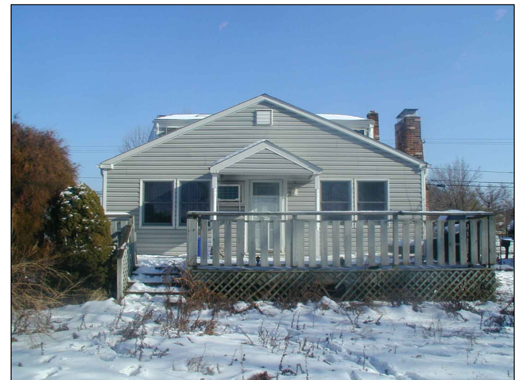
PHOTO VIEW OF DWELLING FROM THE EAST
