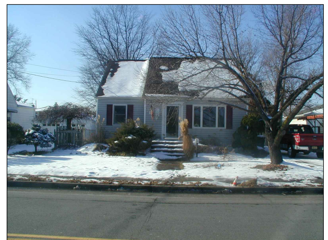
PHOTO VIEW OF DWELLING FROM THE EAST
