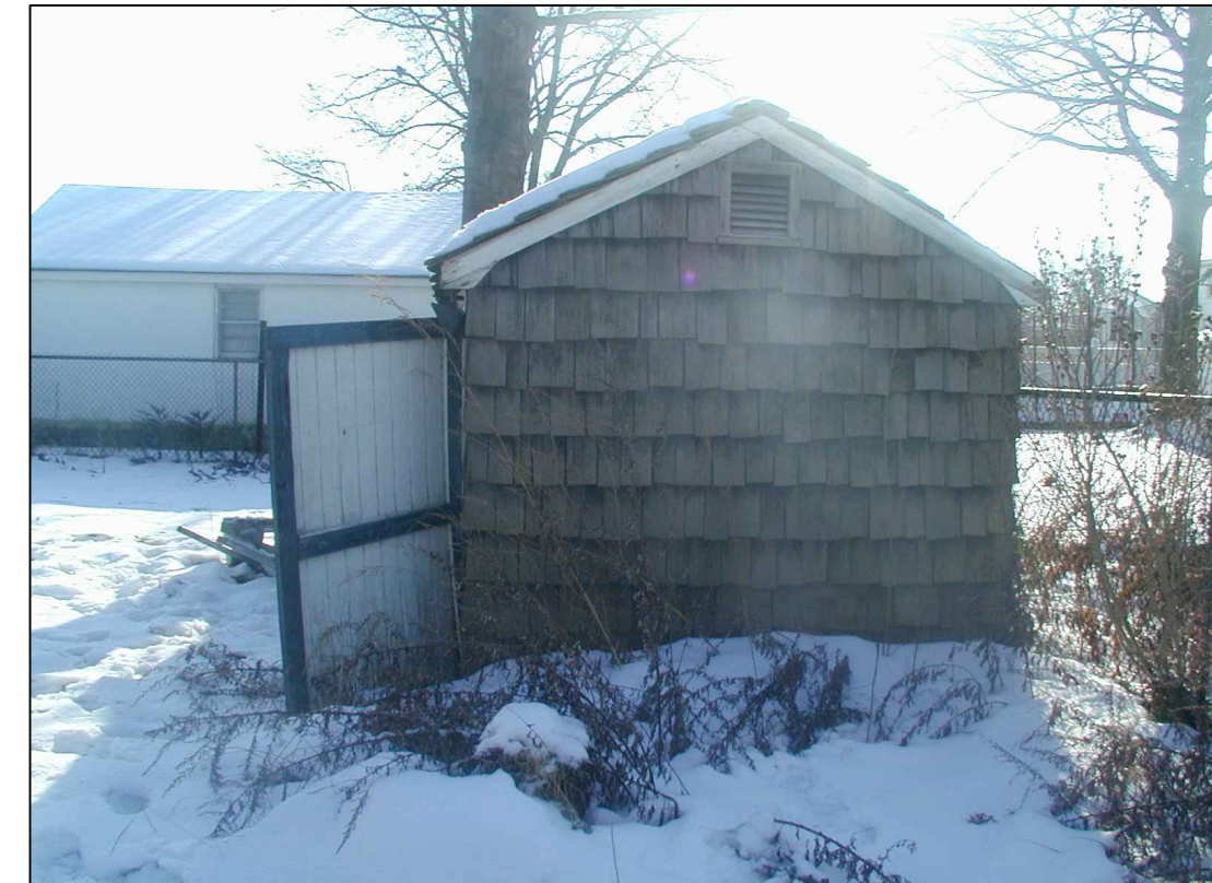
PHOTO VIEW OF SHED FROM THE NORTH
