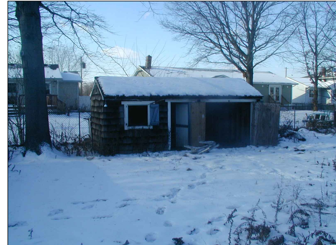
PHOTO VIEW OF SHED FROM THE EAST
