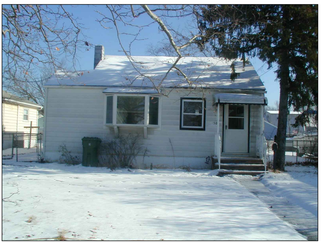
PHOTO VIEW OF DWELLING FROM THE WEST
