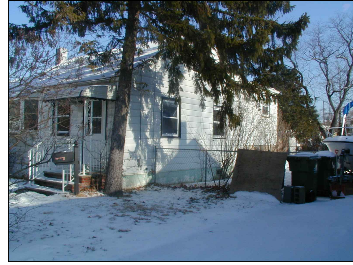
PHOTO VIEW OF DWELLING FROM THE EAST
