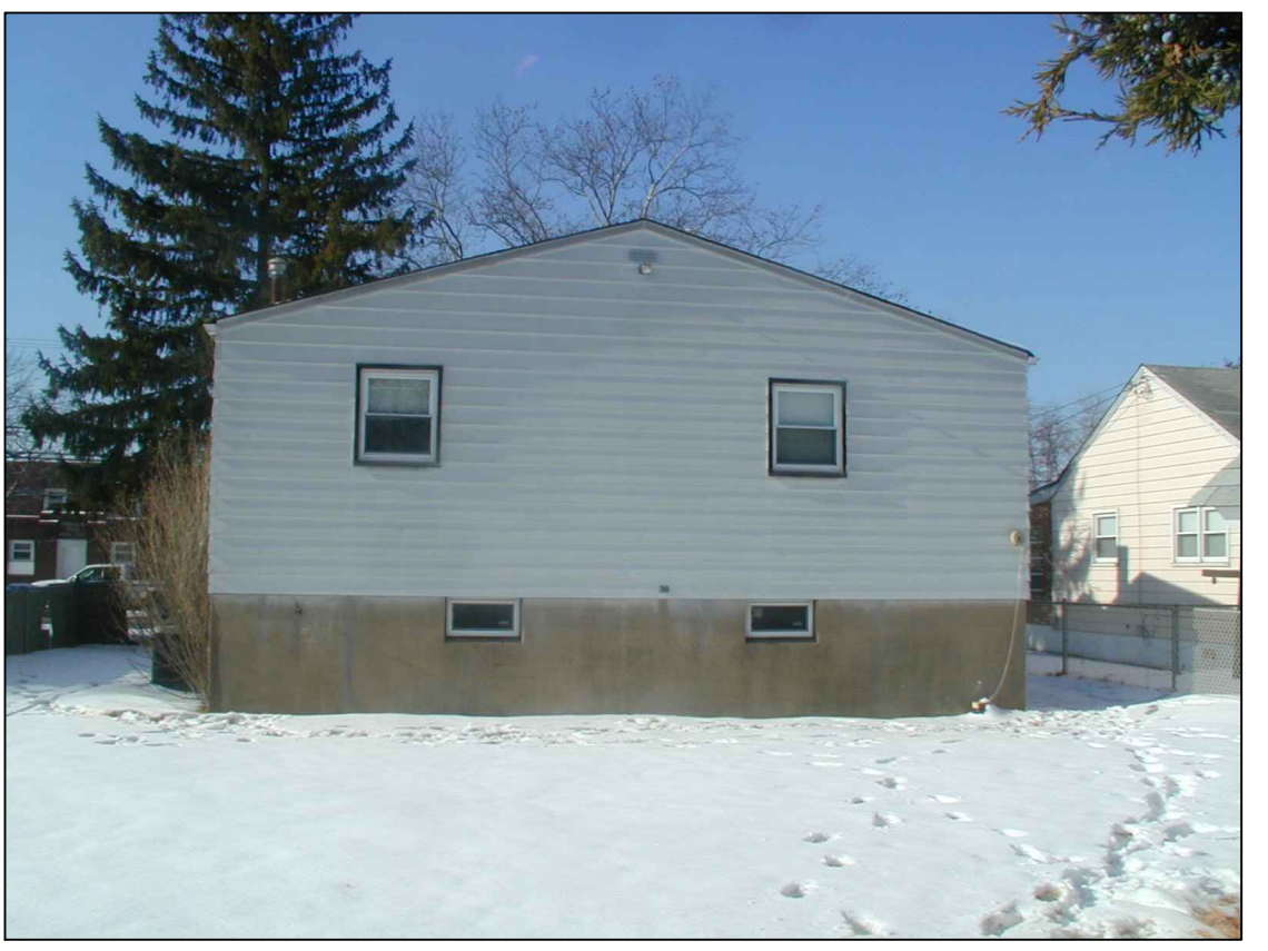
PHOTO VIEW OF DWELLING FROM THE EAST
