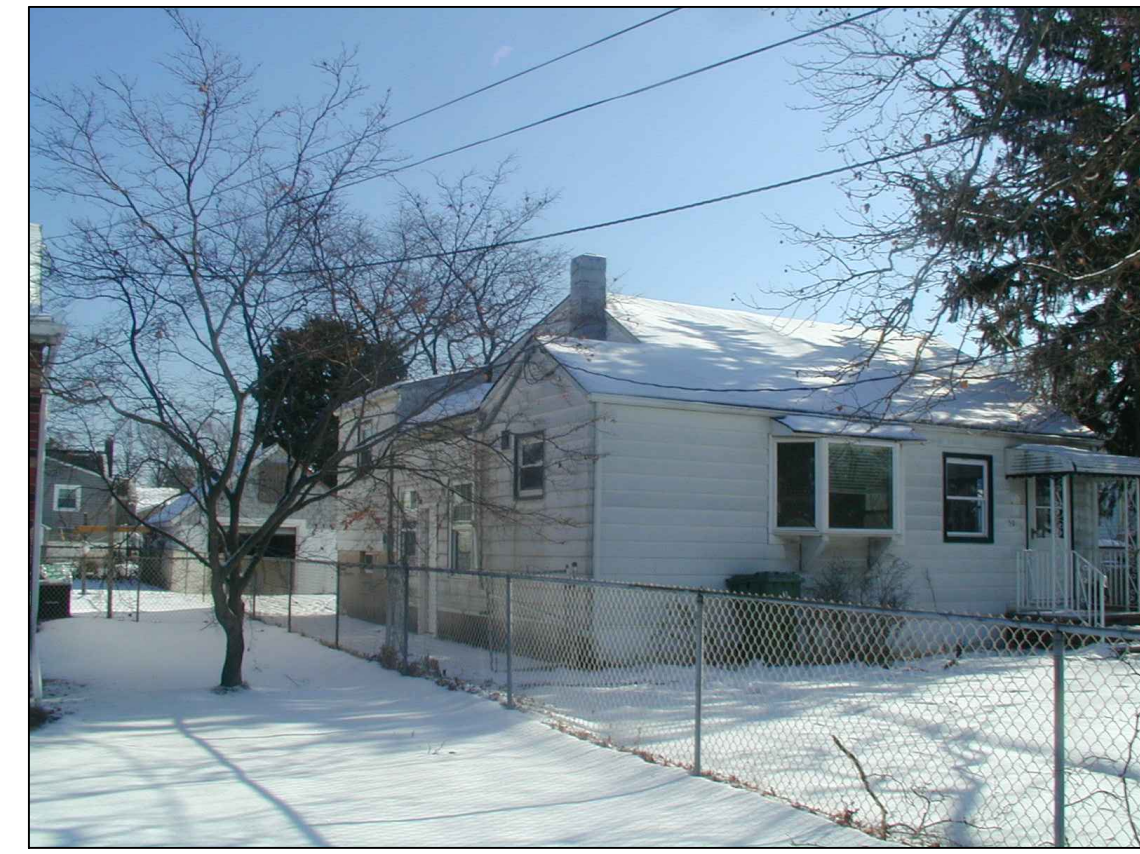
PHOTO VIEW OF DWELLING FROM THE WEST
