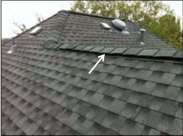
Figure 3. Roofing with ridge vent (source: ABARoofing.net).
