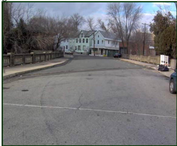
Wall Street Bridge BEFORE
