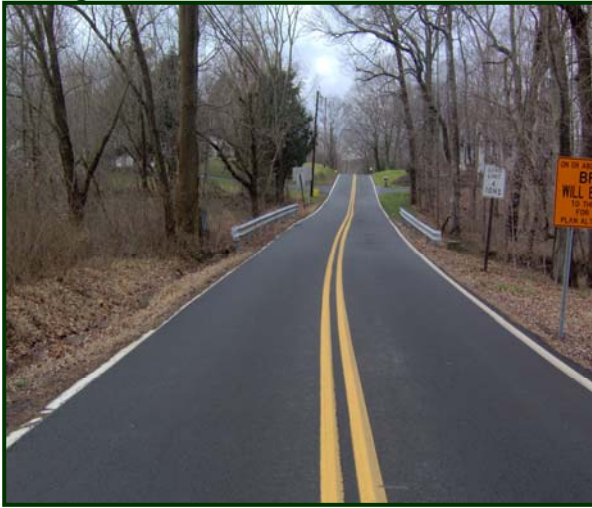
Federal City Road Bridge BEFORE
