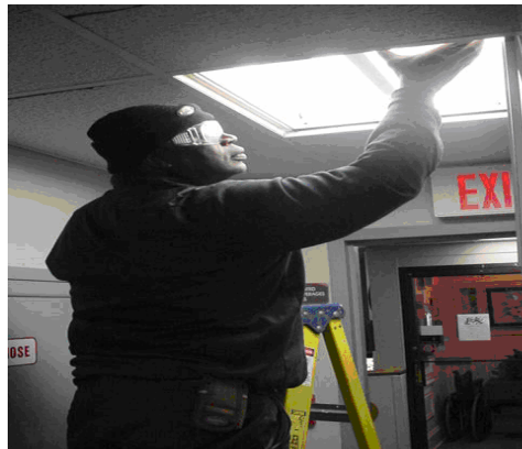
Maintenance Repair Work in Main Terminal
