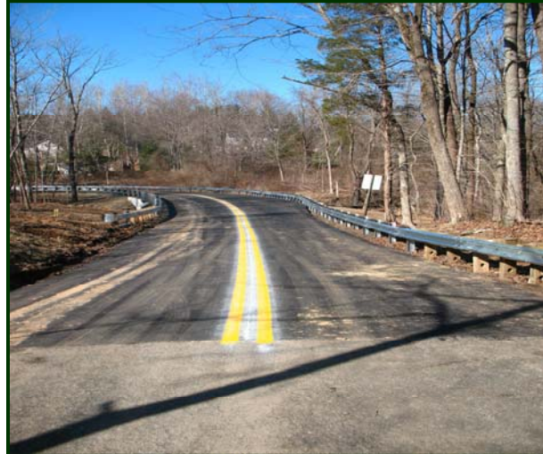
Stony Brook Road Bridge AFTER
