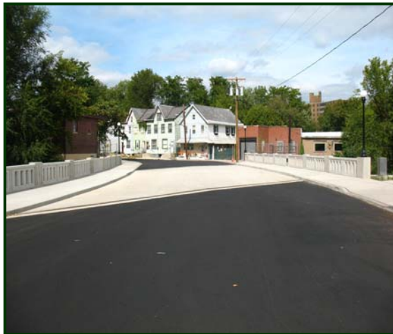
Wall Street Bridge AFTER
