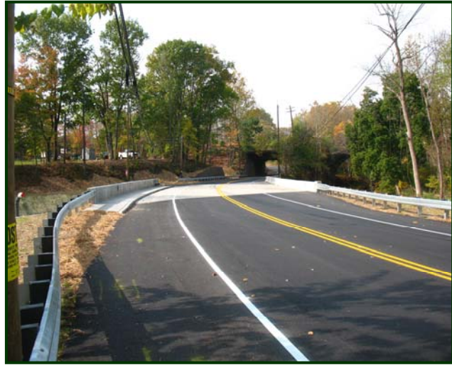
Pennington-Hopewell Road Bridge AFTER
