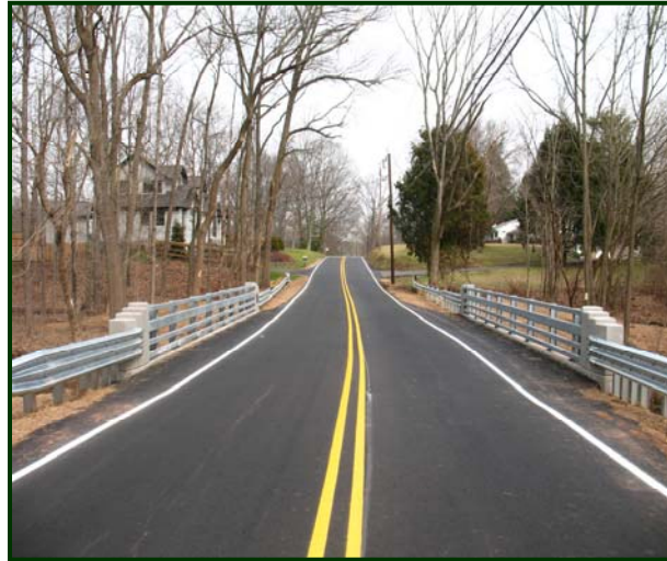
Federal City Road Bridge AFTER
