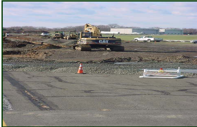
Taxiway A, C, and J Rehabilitation Project
