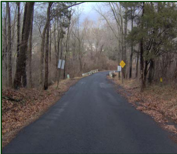
Stony Brook Road Bridge BEFORE
