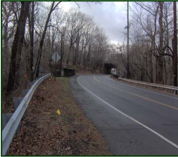
Pennington-Hopewell Road Bridge BEFORE
