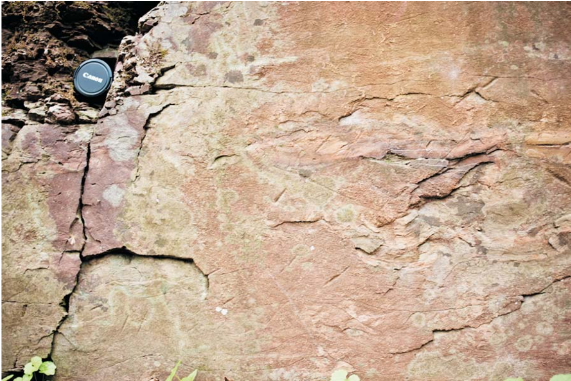
Plate 8. Evidence of pick and chisel marks along quarry face, looking west.
