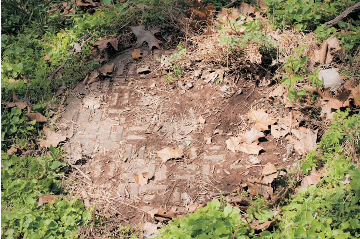
Plate 5. Manhole cover for sewer line crossing Jacob's Creek.
