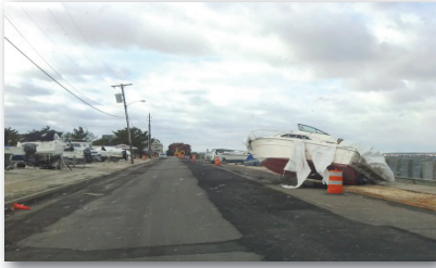
Repair, replacement or relocation of damaged infrastructure is also a priority for use of these dollars.
