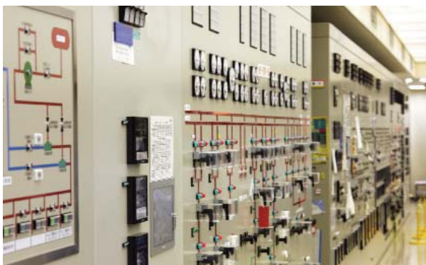
Figure D-5 Substation Control Room
