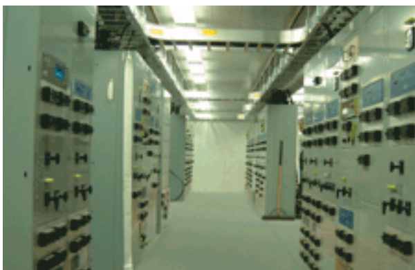
Figure D-4 Substation Control Room
