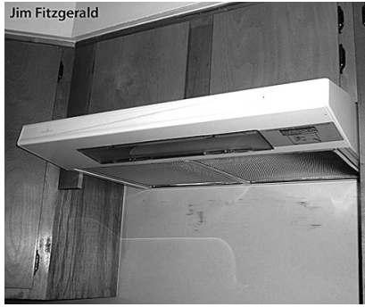
Advanced 4-speed range fan: Lower speeds for continuous ventilation and higher ones for spot ventilation.
