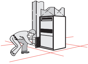
Panel filter installed in filter slot in return plenum
