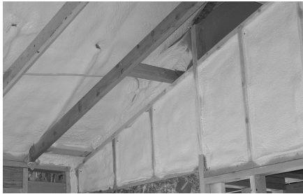
Foam insulated roof of vault: Vaults can be filled with stabilized insulation or their roof decks can be sprayed with foam.
