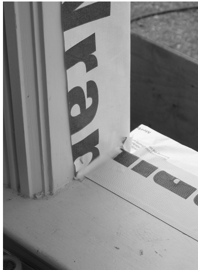
Flashing an existing window frame: Wrap the water-resistant barrier from the outside to the interior of the window frame so that any penetrating moisture will drain out without soaking into the wood.
