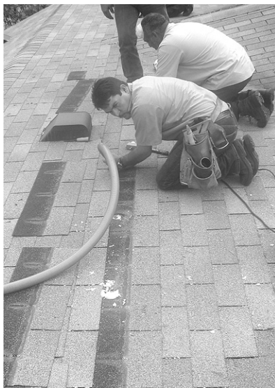
Blowing from the roof deck: Technicians remove a row of shingles, drill, and blow fiberglass into this vaulted roof cavity.
