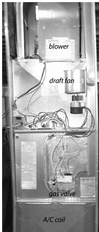
Fan-assisted, mid-efficiency mobile home furnace: The draft fan draws outdoor air into the combustion chamber to feed combustion.
