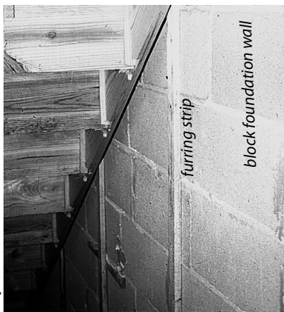
Furring strip leakage: Unsheathed furring strips behind a stairway opens a channel between basement and attic at a party wall between townhouses.
