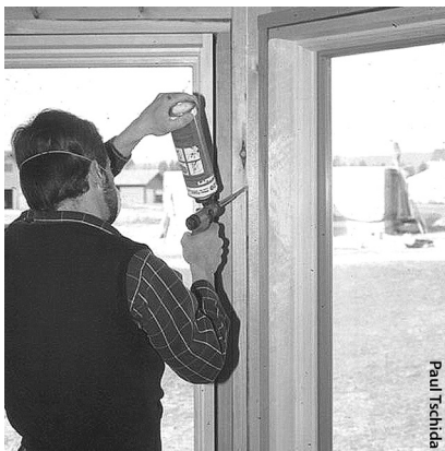
One-part foam: A contractor uses an applicator gun to seal spaces between framing members and around windows.
