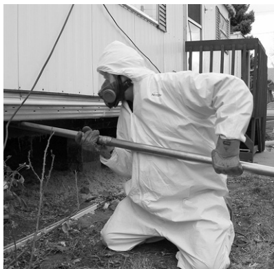
Blowing a floor through the belly: The contractor inserts a rigid fill tube through the belly to blow insulation into the floor cavity and underbelly.
