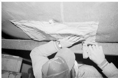
Patching a flexible belly: The technician uses both adhesive and stitch staples to fasten a patch.
