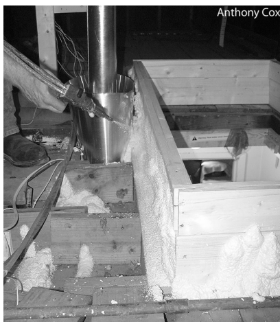
Two-part foam: A contractor air seals and insulates around an attic hatch dam with two-part spray foam.
