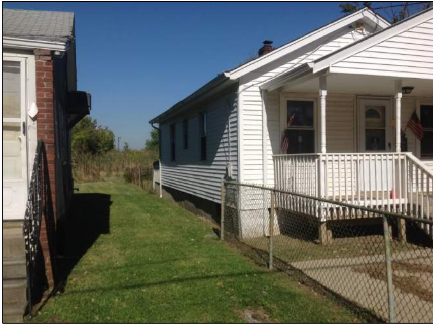
Photo 3: Left Side of House
