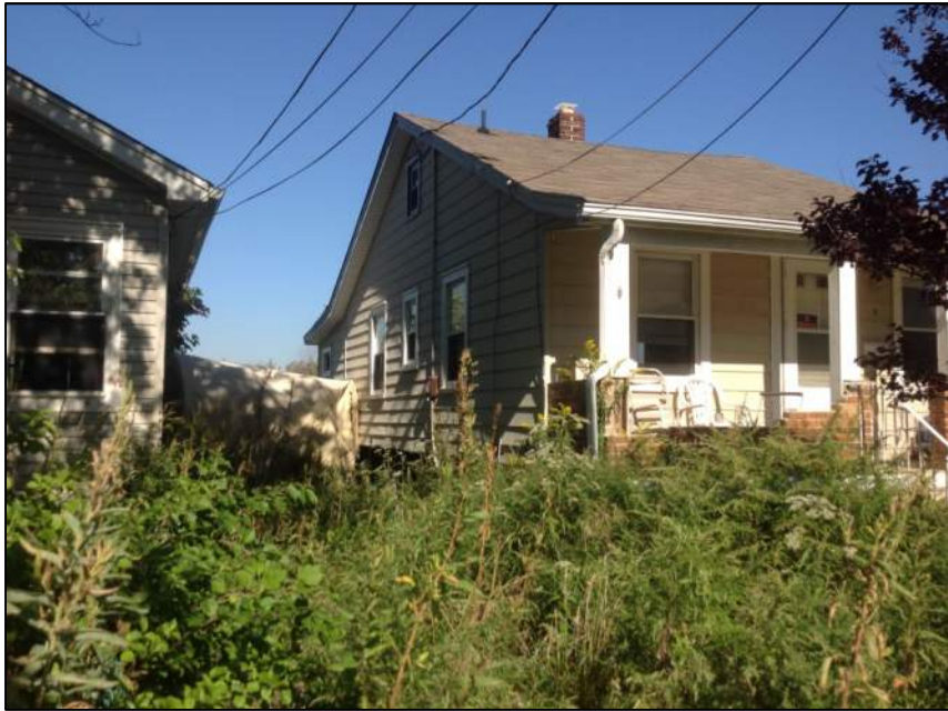
Photo 3: Left Side of House
