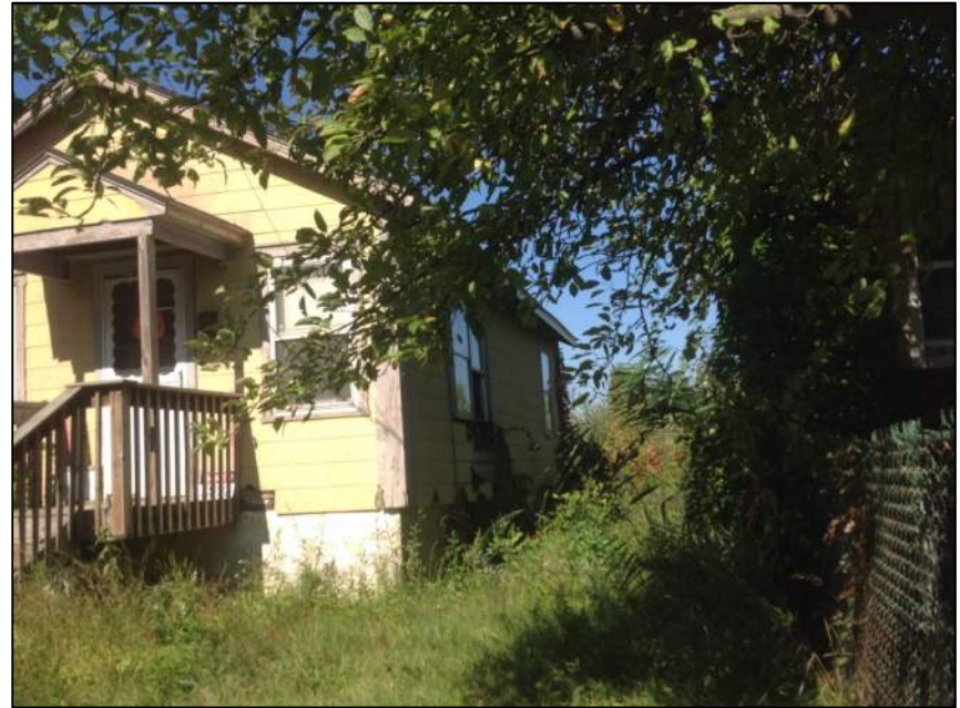
Photo 4: Right Side of House
