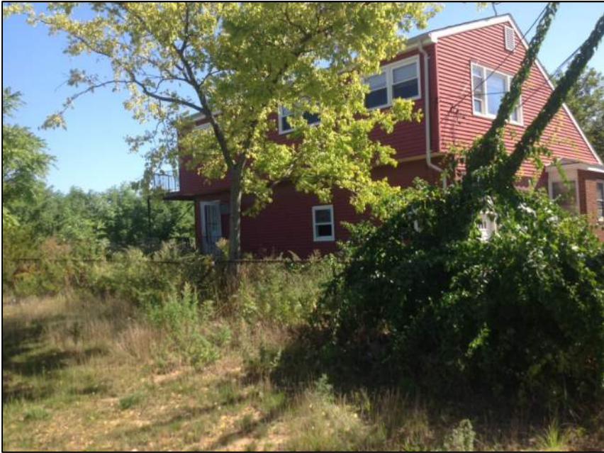
Photo 3: Left Side of House
