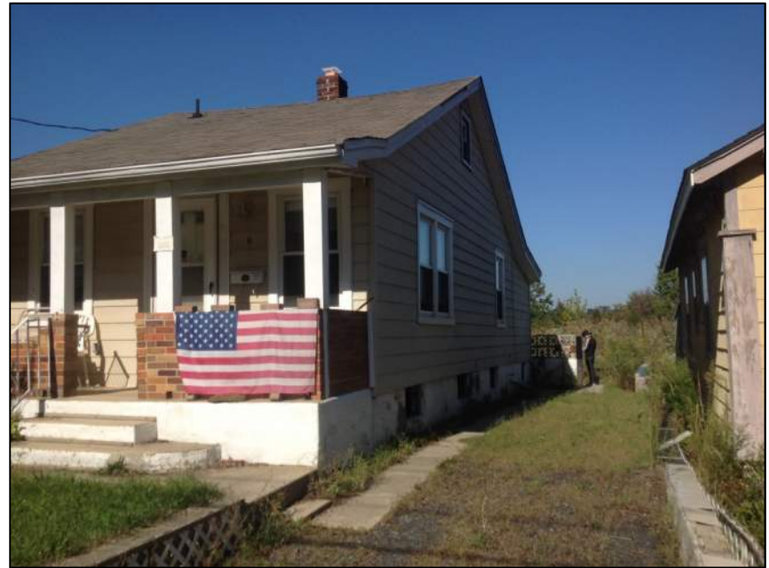
Photo 4: Right Side of House
