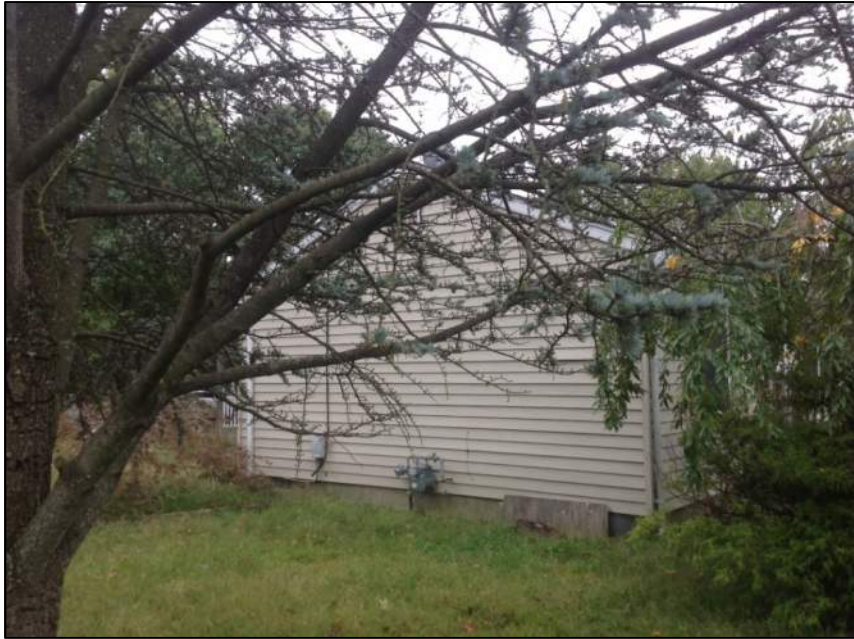
Photo 3: Left Side of House
