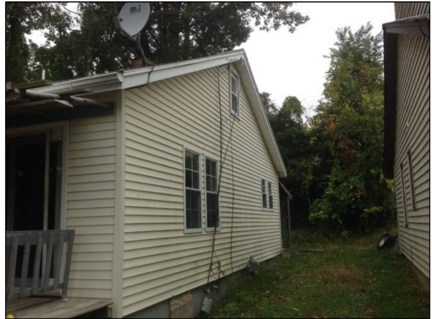
Photo 4: Right Side of House
