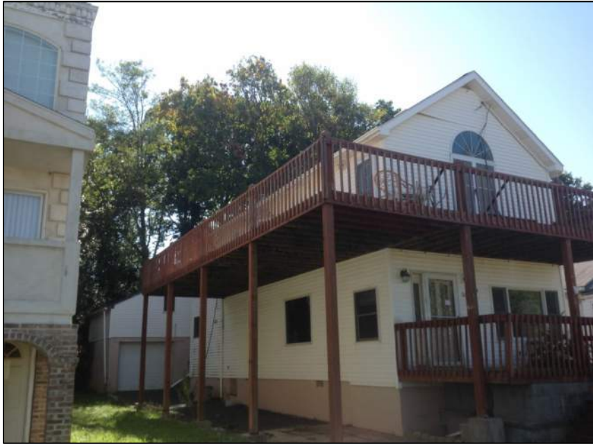
Photo 3: Left Side of House
