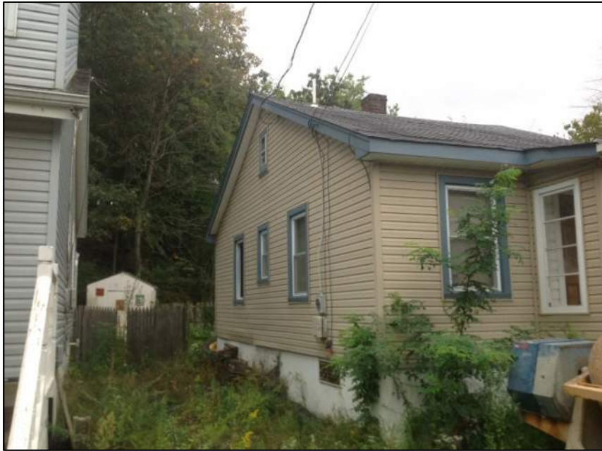
Photo 3: Left Side of House
