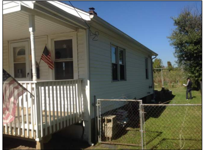
Photo 4: Right Side of House
