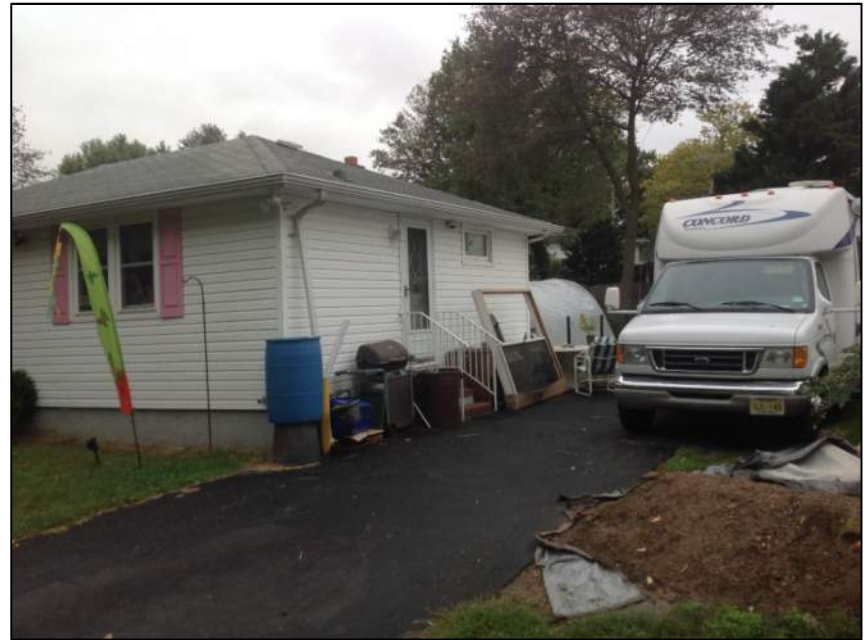
Photo 4: Right Side of House
