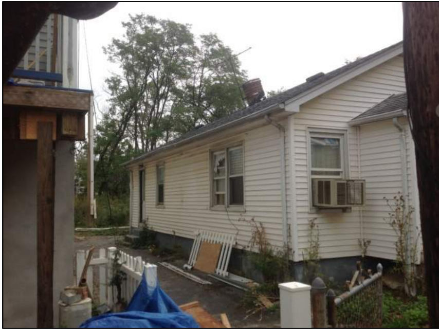
Photo 3: Left Side of House
