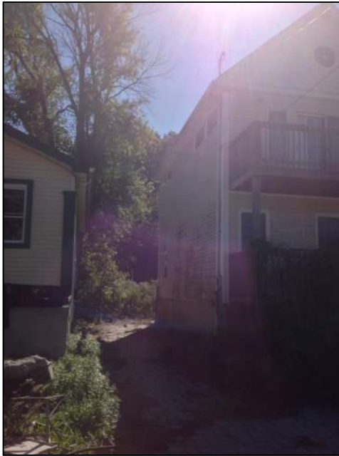
Photo 3: Left Side of House
