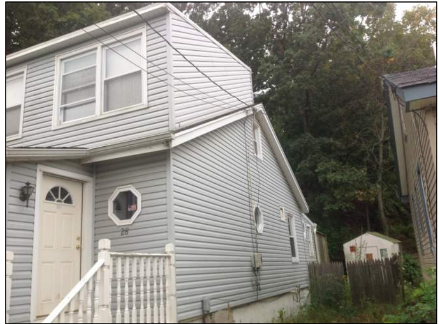
Photo 4: Right Side of House
