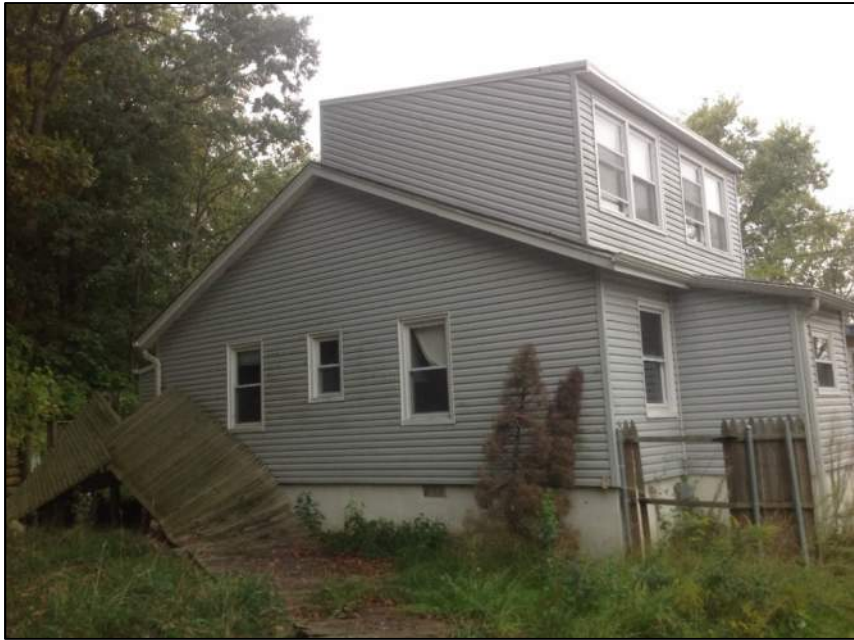
Photo 3: Left Side of House
