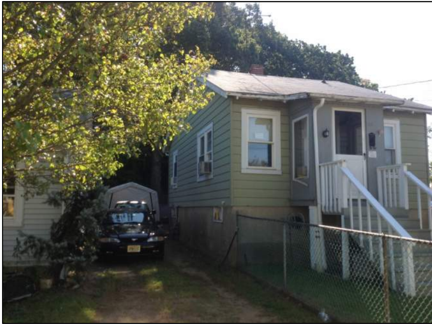
Photo 3: Left Side of House
