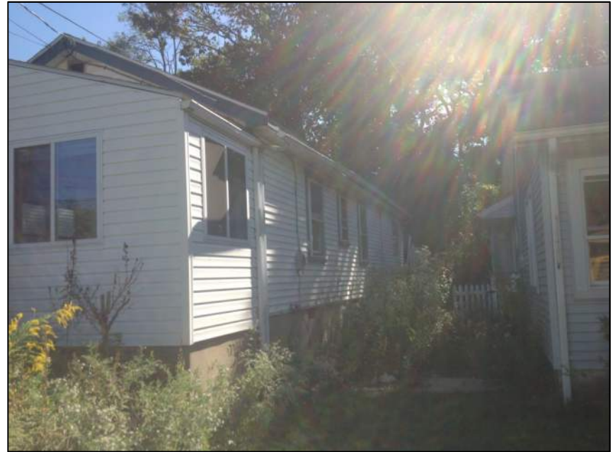
Photo 4: Right Side of House
