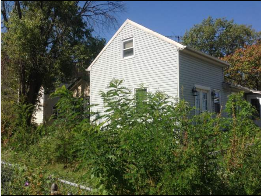
Photo 3: Left Side of House
