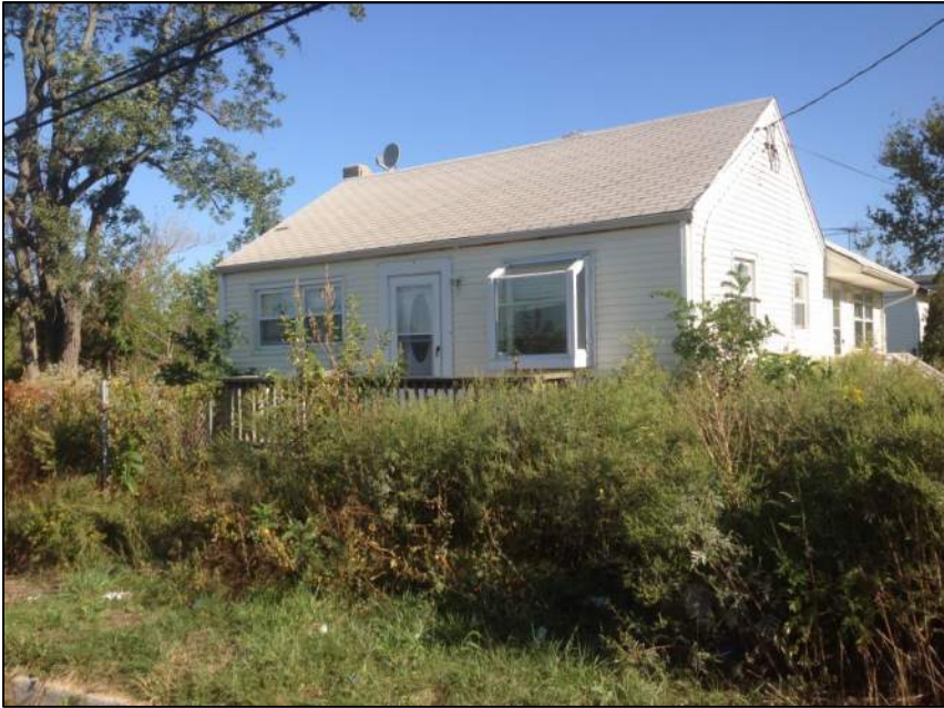
Photo 3: Left Side of House
