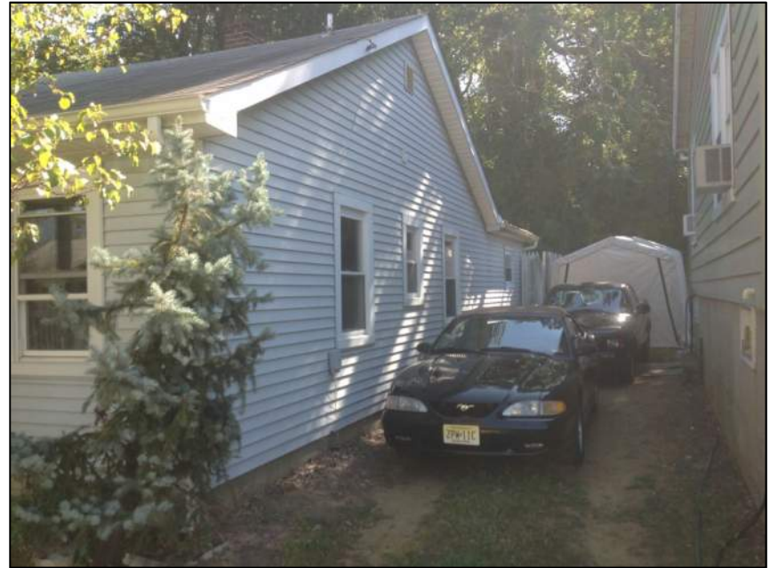
Photo 4: Right Side of House
