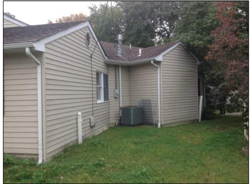
Photo 4: Right Side of House
