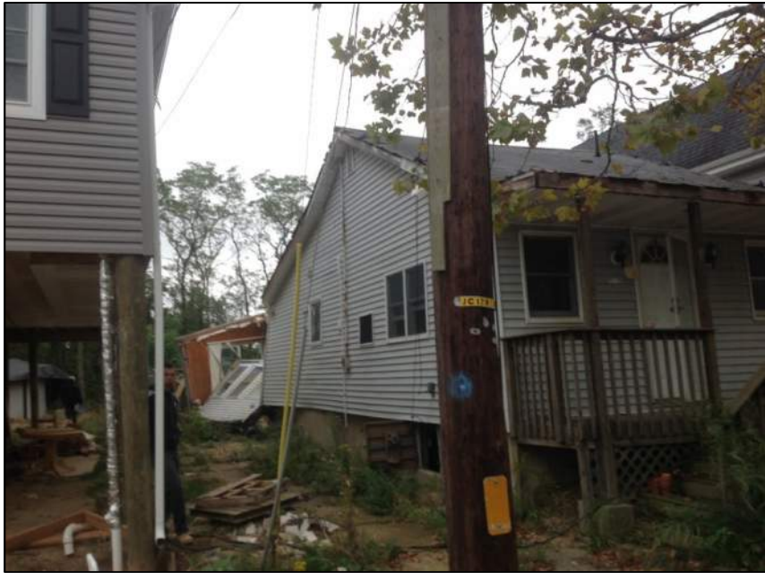
Photo 3: Left Side of House
