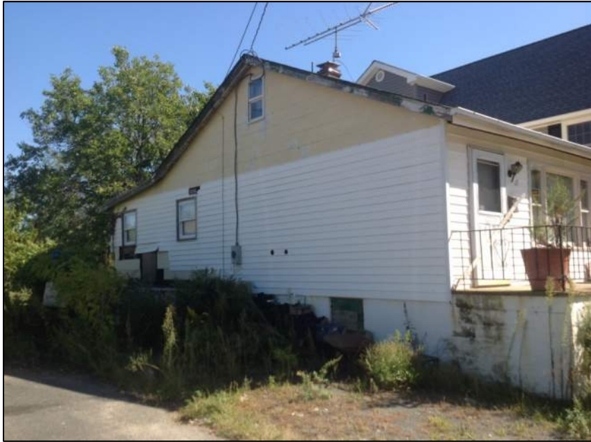
Photo 3: Left Side of House
