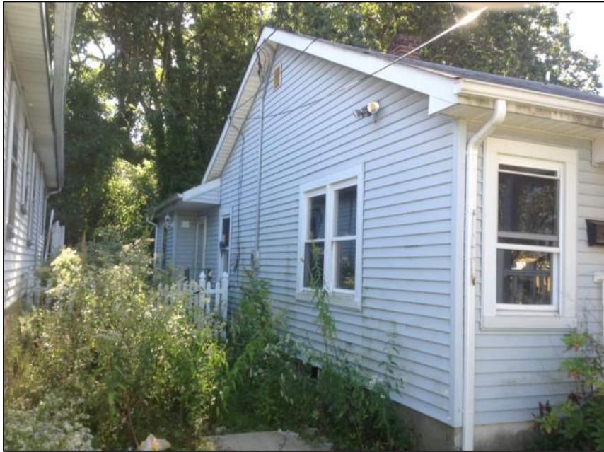
Photo 3: Left Side of House
