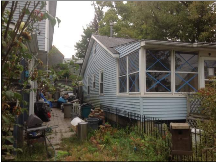
Photo 3: Left Side of House
