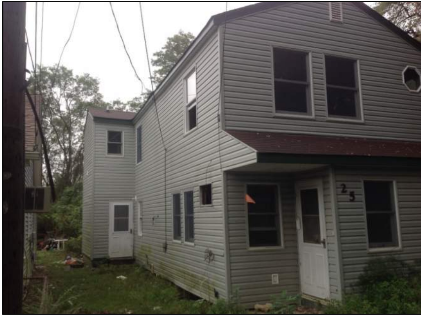
Photo 3: Left Side of House
