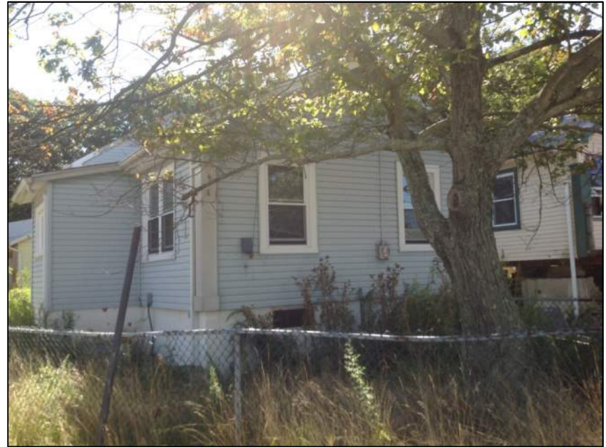
Photo 4: Right Side of House
