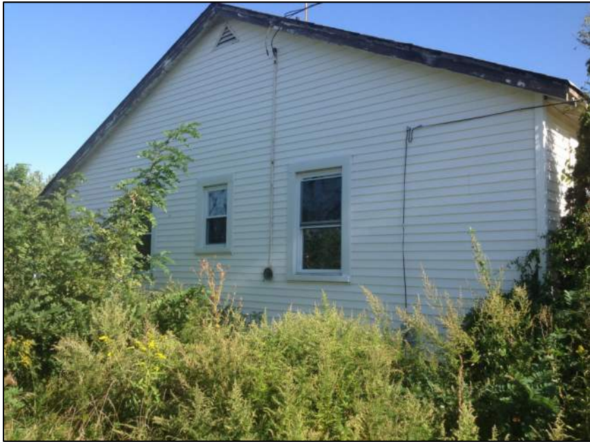
Photo 3: Left Side of House
