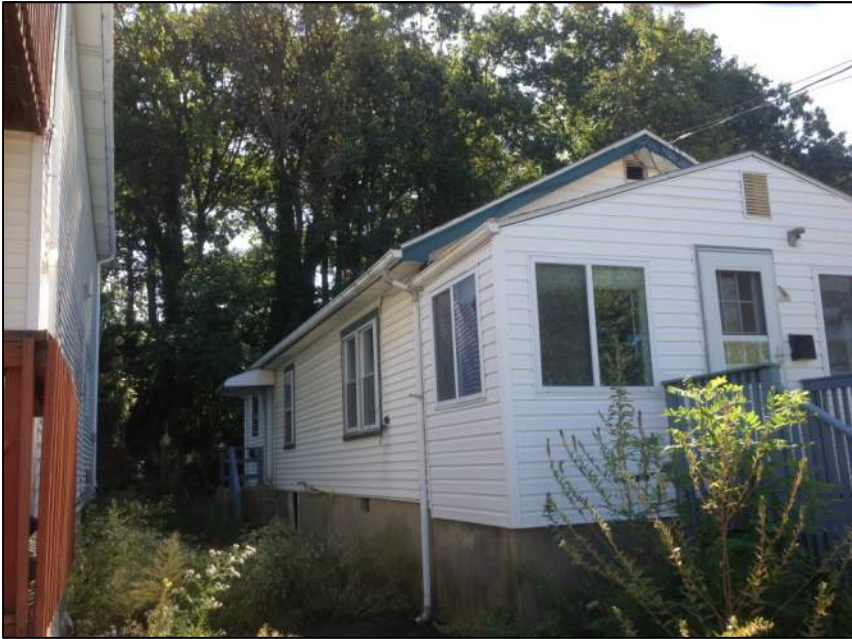
Photo 3: Left Side of House
