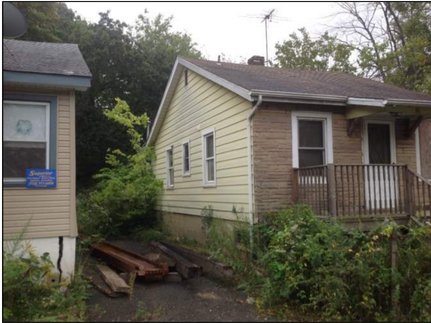
Photo 3: Left Side of House
