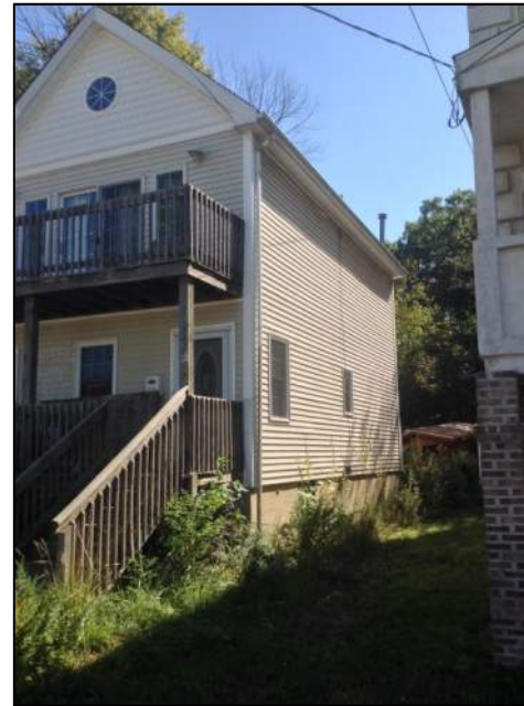
Photo 4: Right Side of House
