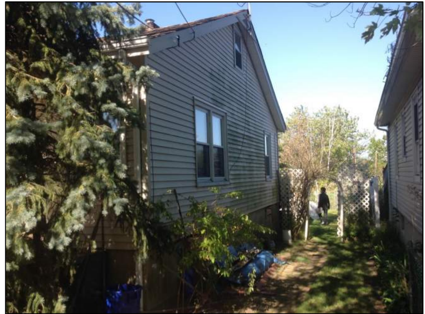
Photo 4: Right Side of House
