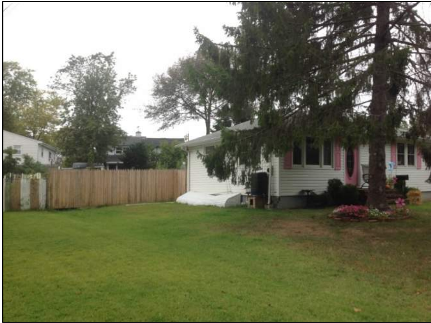
Photo 3: Left Side of House
