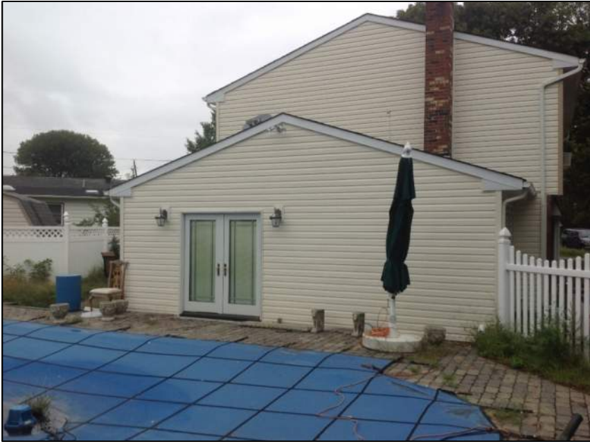
Photo 3: Left Side of House
