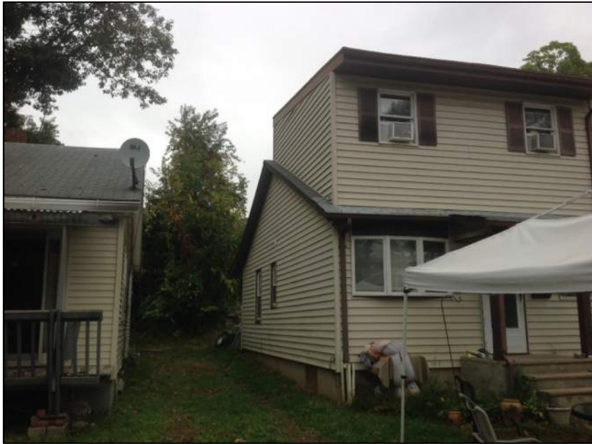
Photo 3: Left Side of House
