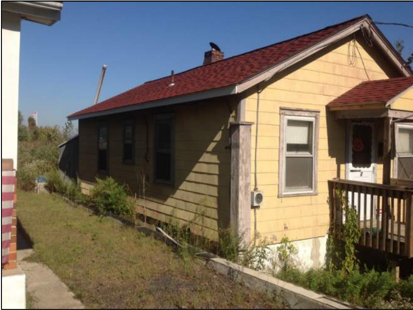
Photo 3: Left Side of House
