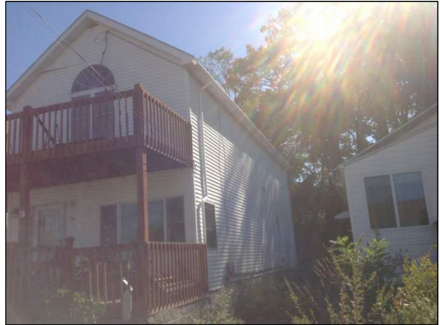
Photo 4: Right Side of House
