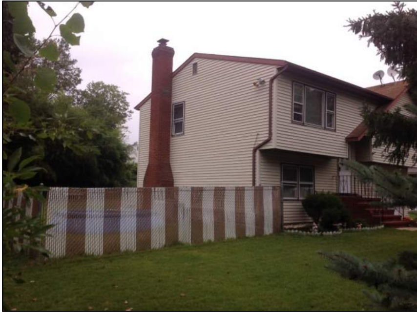
Photo 3: Left Side of House
