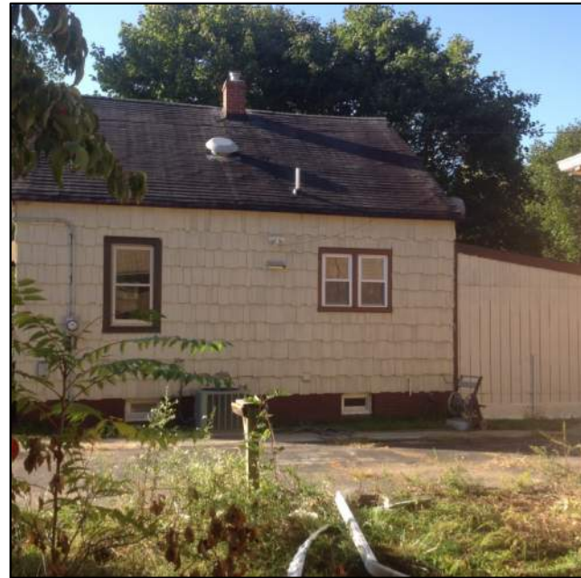
Photo 4: Right Side of House
