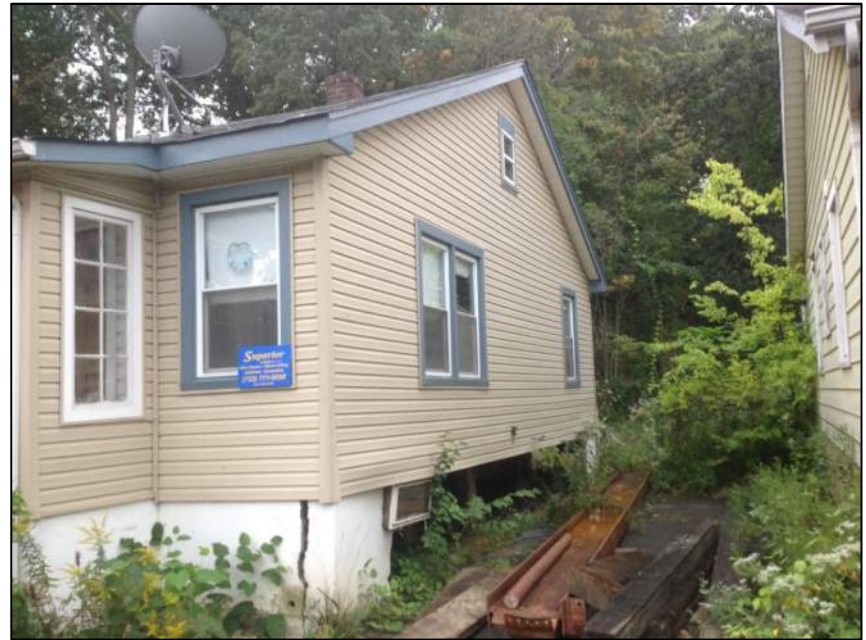
Photo 4: Right Side of House
