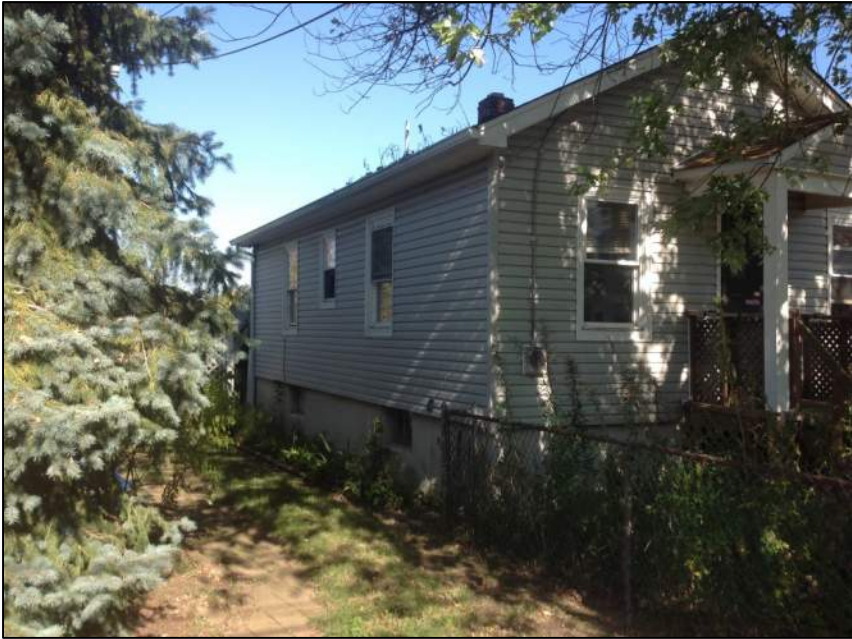
Photo 3: Left Side of House
