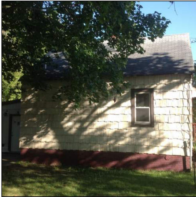
Photo 3: Left Side of House
