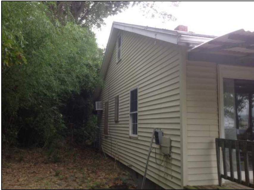
Photo 3: Left Side of House
