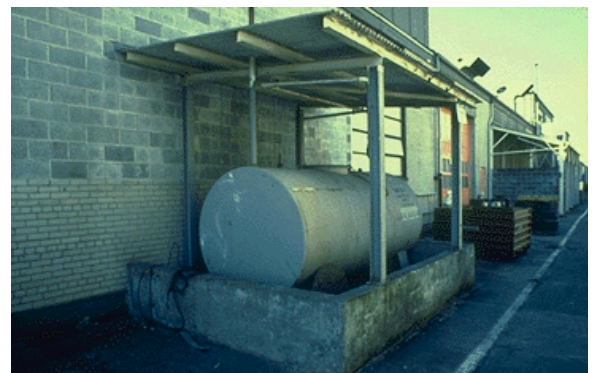
Covered AST with secondary containment
