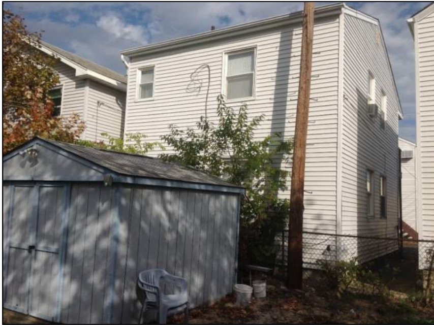
Photo 7: Rear View – Building No. 2
