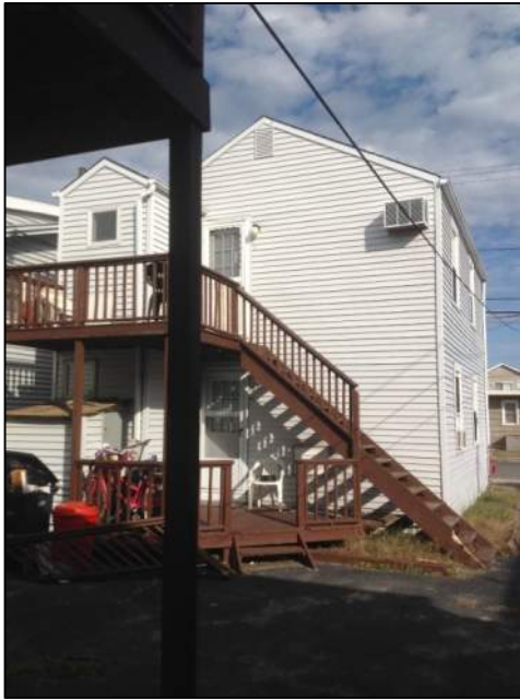
Photo 3: Rear View – Building No. 1
