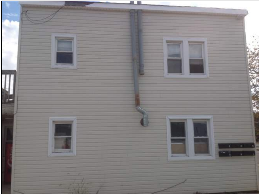
Photo 3: Left View – Building No. 1
