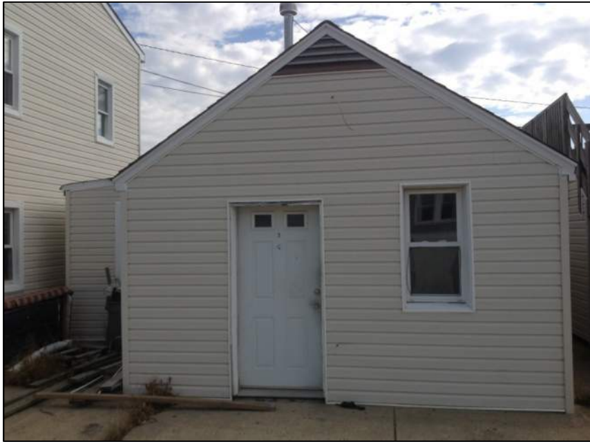
Photo 5: Front View – Building No. 2
