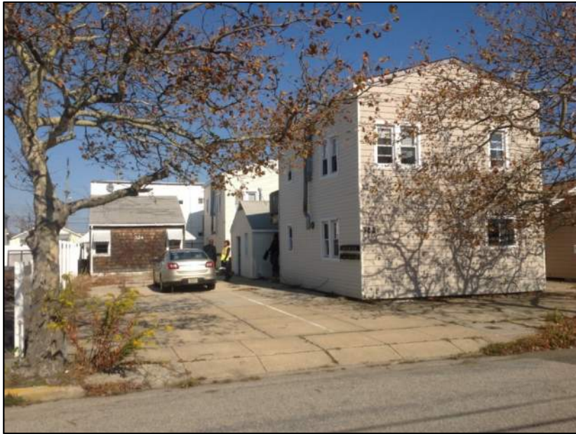
Photo 1: Front View – Overall Site
