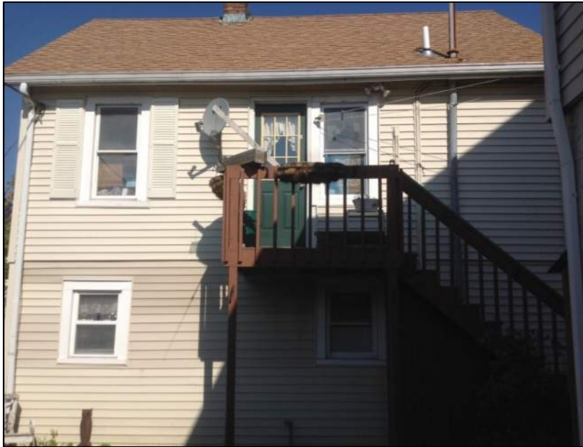
Photo 7: Left View – Building No. 2
