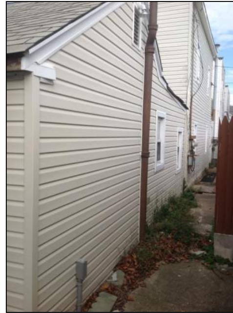
Photo 6: Rear View – Building No. 2
