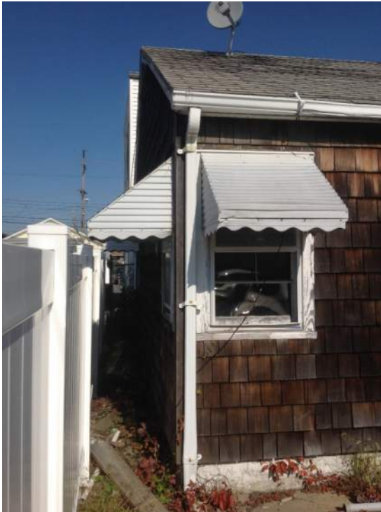
Photo 15: Left View – Building No. 4
