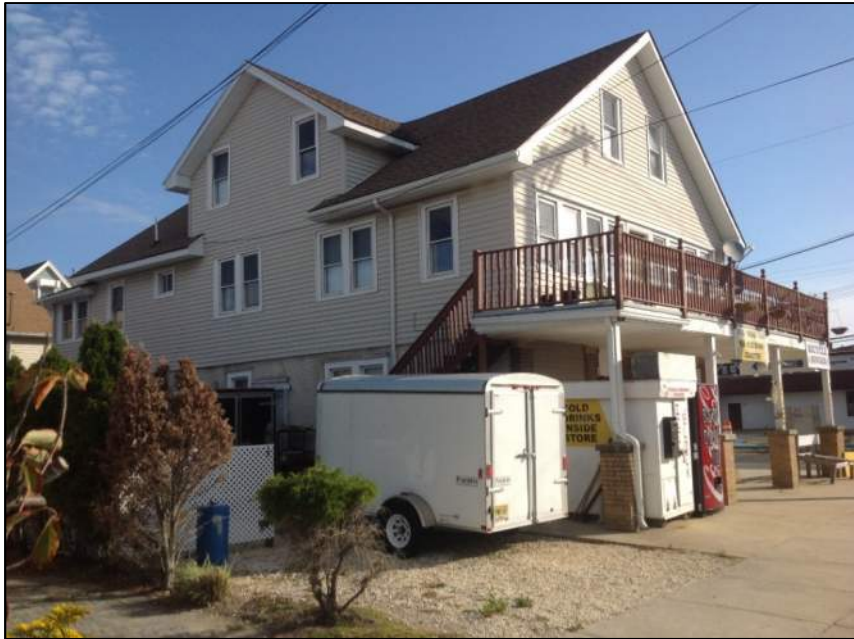
Photo 3: Left View – Building No. 1
