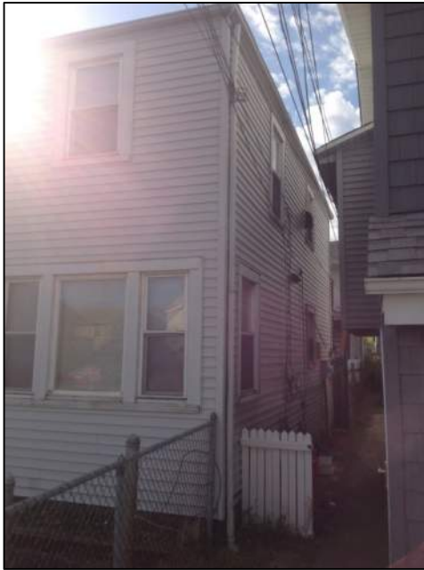
Photo 5: Right View – Building No. 1
