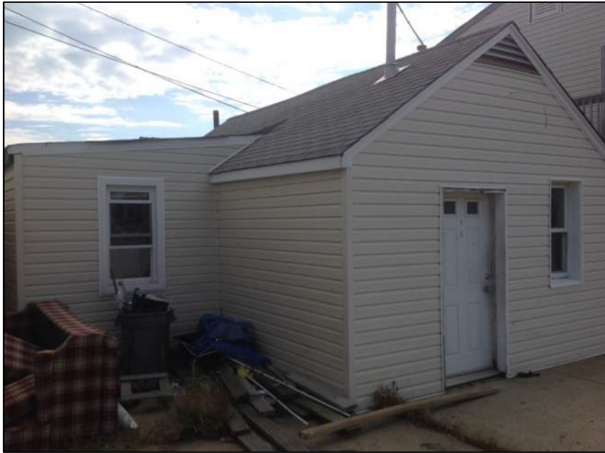
Photo 7: Left View – Building No. 2
