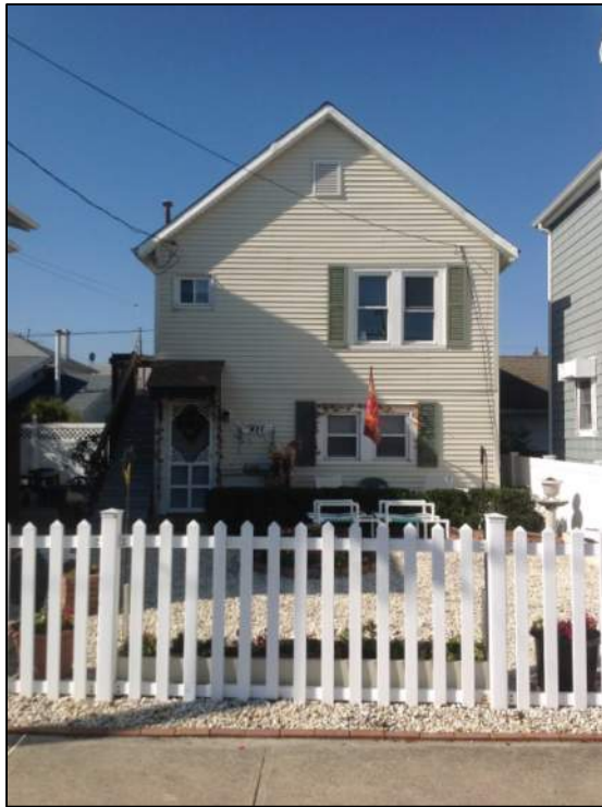
Photo 5: Front View – Building No. 2
