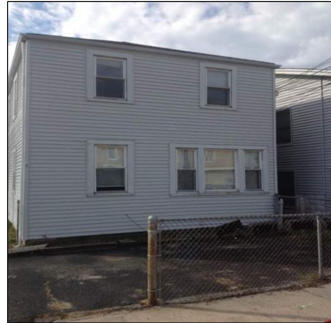
Photo 2: Front View – Building No. 1
