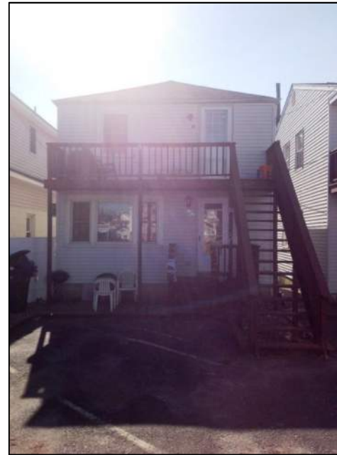
Photo 10: Front View – Building No. 3
