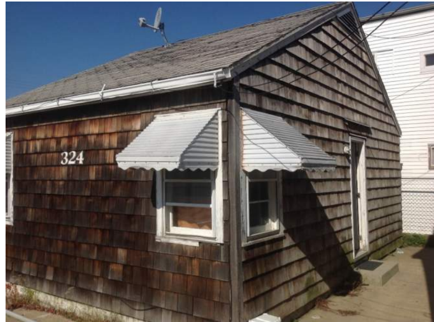
Photo 16: Right View – Building No. 4
