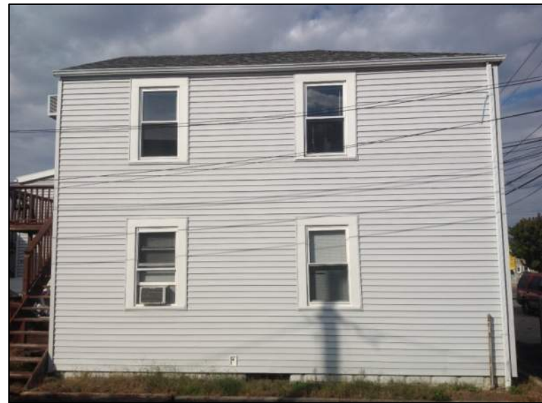
Photo 4: Left View – Building No. 1
