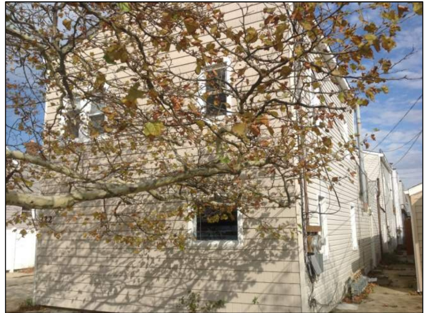
Photo 4: Right View– Building No. 1
