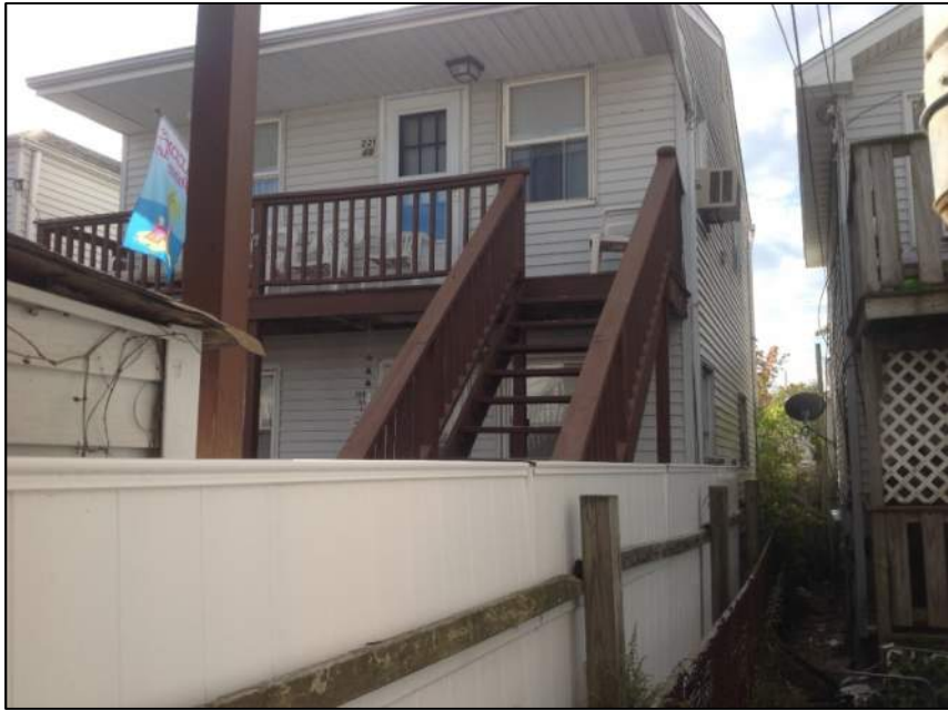
Photo 9: Right View – Building No.2
