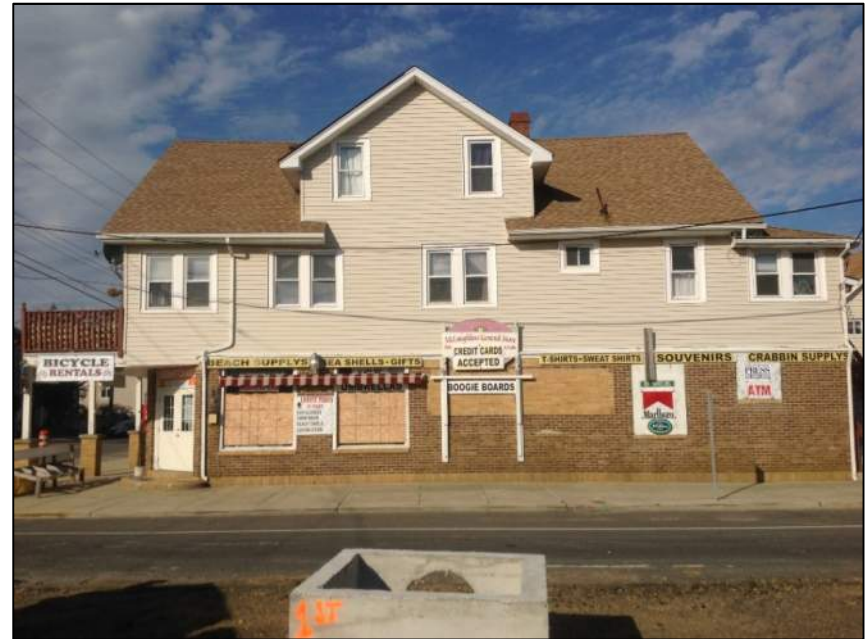
Photo 4: Right View – Building No. 1
