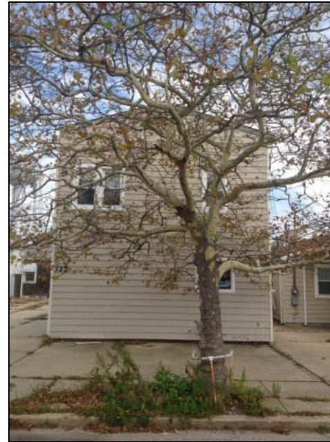
Photo 2: Front View – Building No. 1
