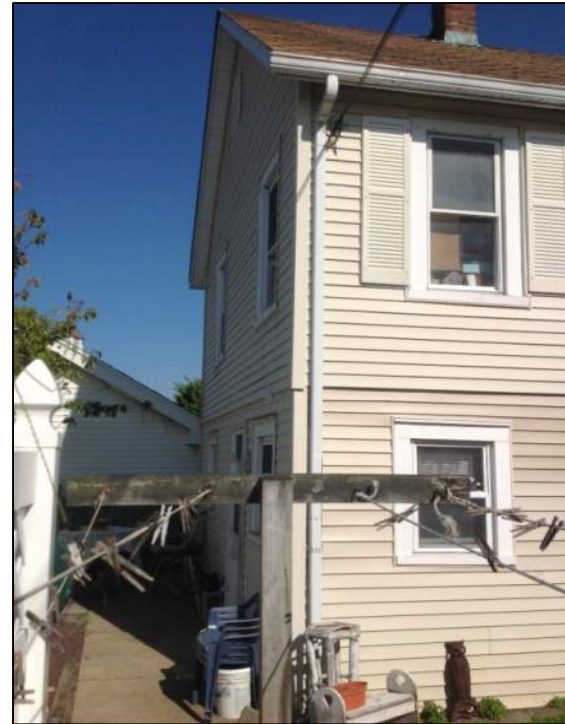
Photo 6: Back View – Building No. 2
