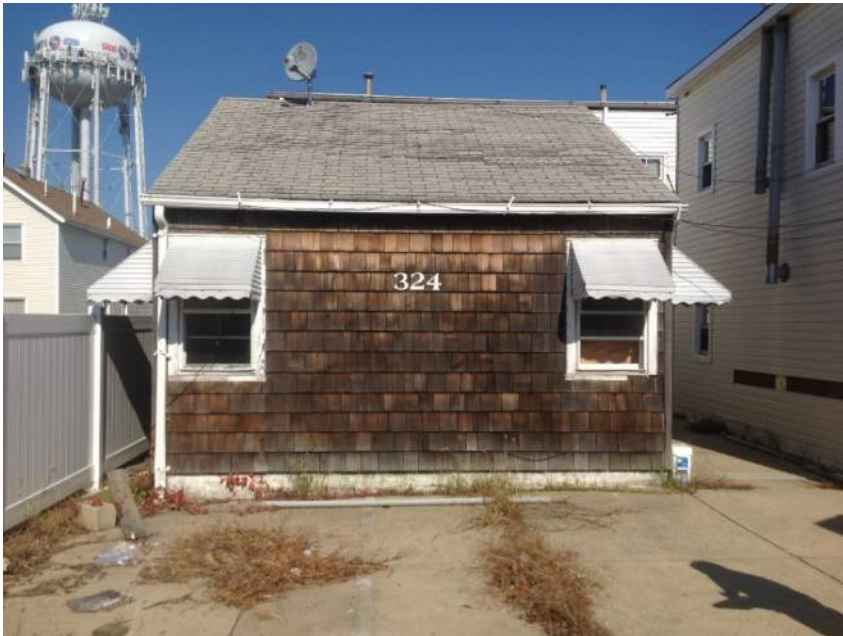
Photo 13: Front View – Building No. 4
