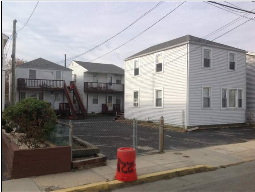
Photo 1: Front View – Overall Site
