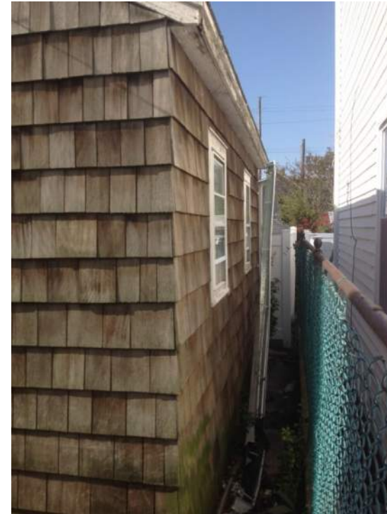
Photo 14: Rear View – Building No. 4
