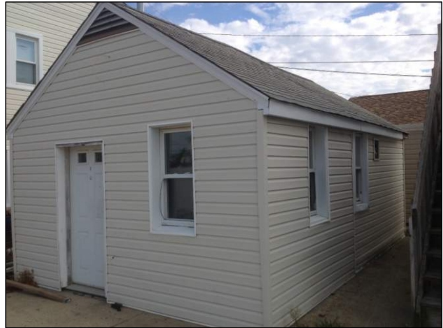
Photo 8: Right View – Building No. 2
