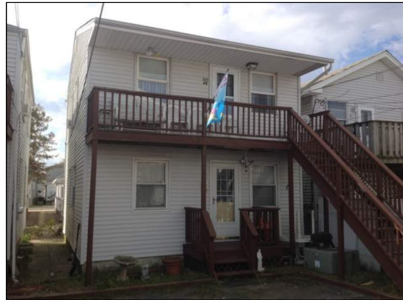
Photo 6: Front View – Building No. 2
