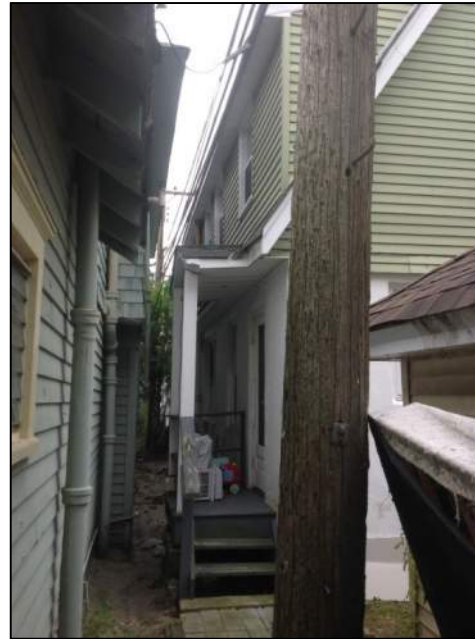
Photo 7: Rear View – Building No.2
