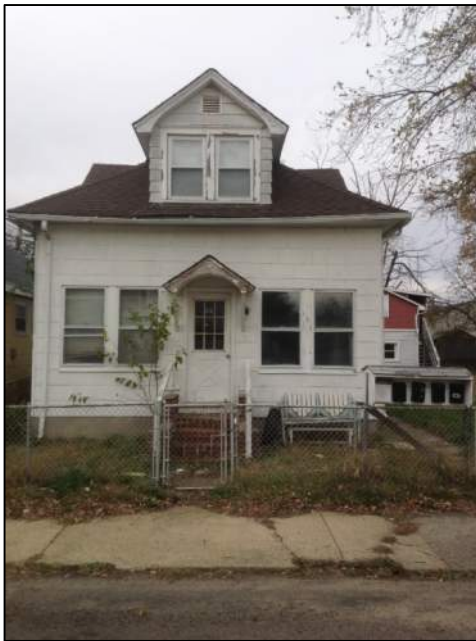
Photo 3: Front View – Building No.1
