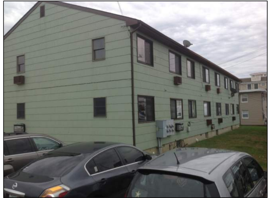
Photo 4: Rear View – Building No.1
