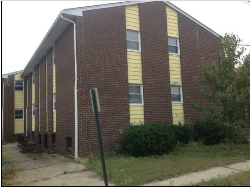
Photo 5: Left View – Building No.1
