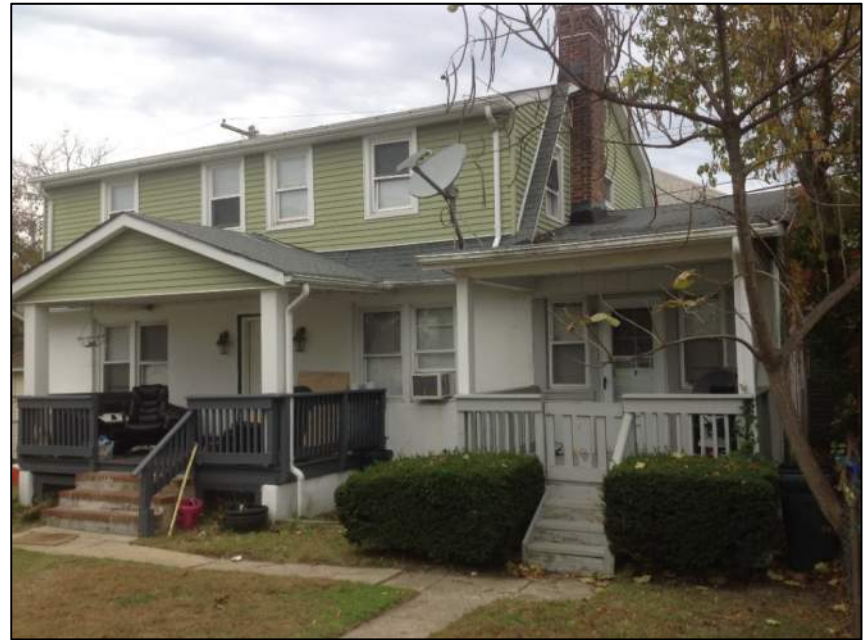
Photo 9: Right View – Building No.2
