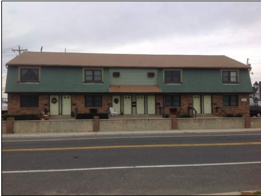
Photo 3: Front View – Building No.1
