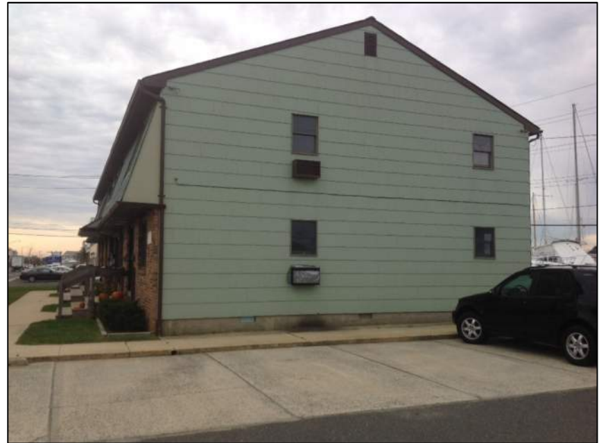
Photo 6: Right View – Building No.1
