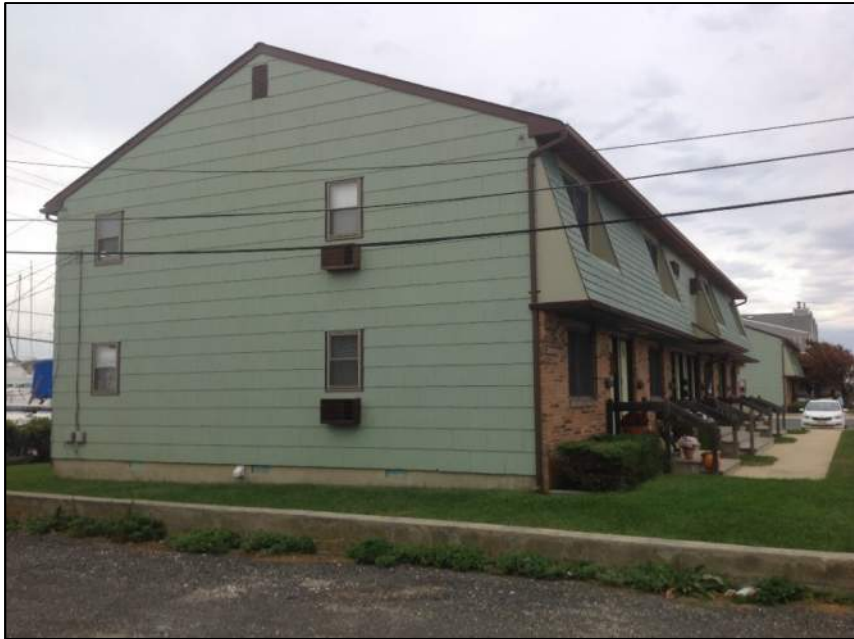
Photo 5: Left View – Building No.1
