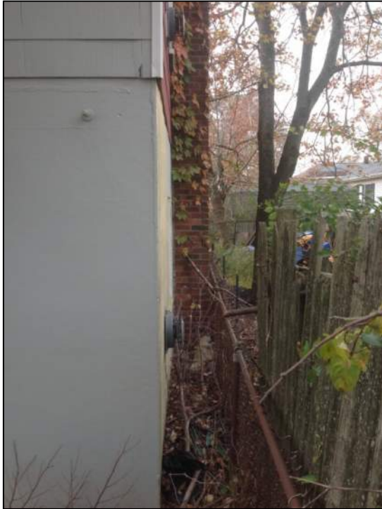
Photo 11: Rear View – Building No.2
