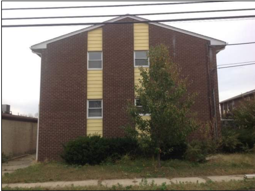
Photo 3: Front View – Building No.1
