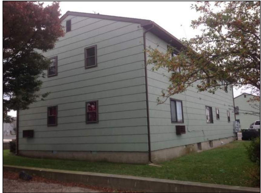
Photo 8: Rear View – Building No.2
