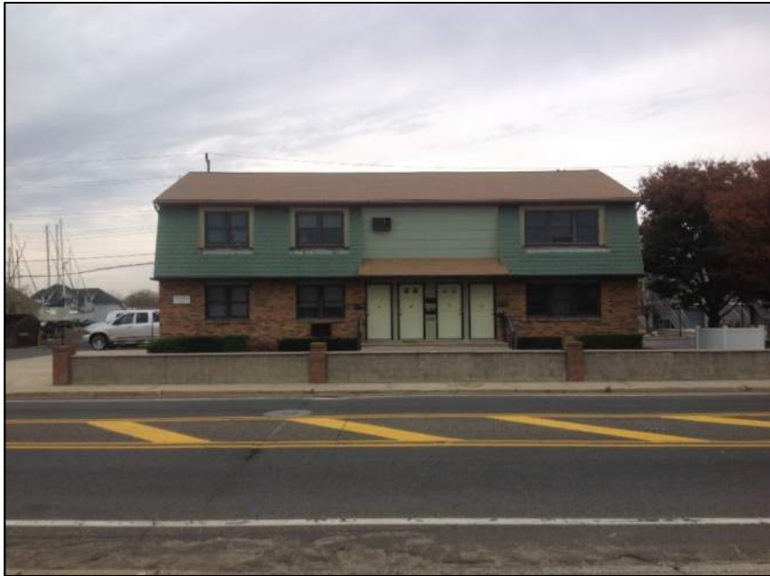
Photo 7: Front View – Building No.2
