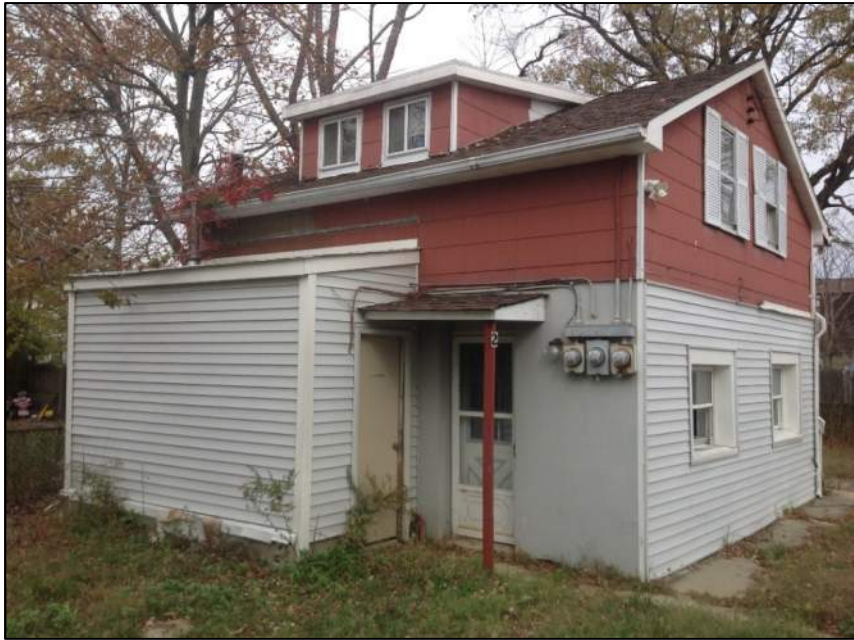
Photo 9: Left View – Building No.2
