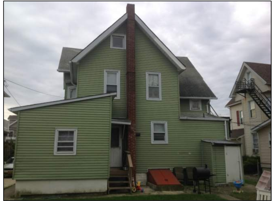
Photo 3: Rear View – Building No.1
