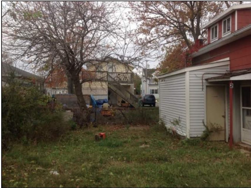
Photo 7: Backyard – Building No.1
