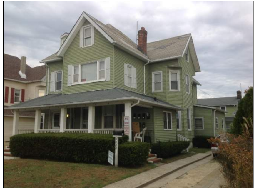
Photo 5: Right View – Building No.1
