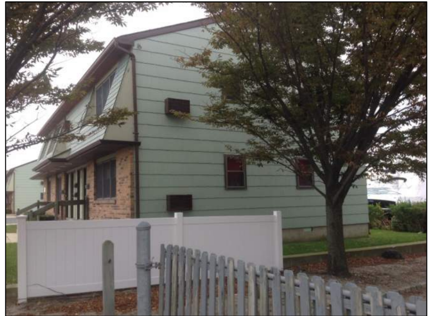
Photo 10: Right View – Building No.2
