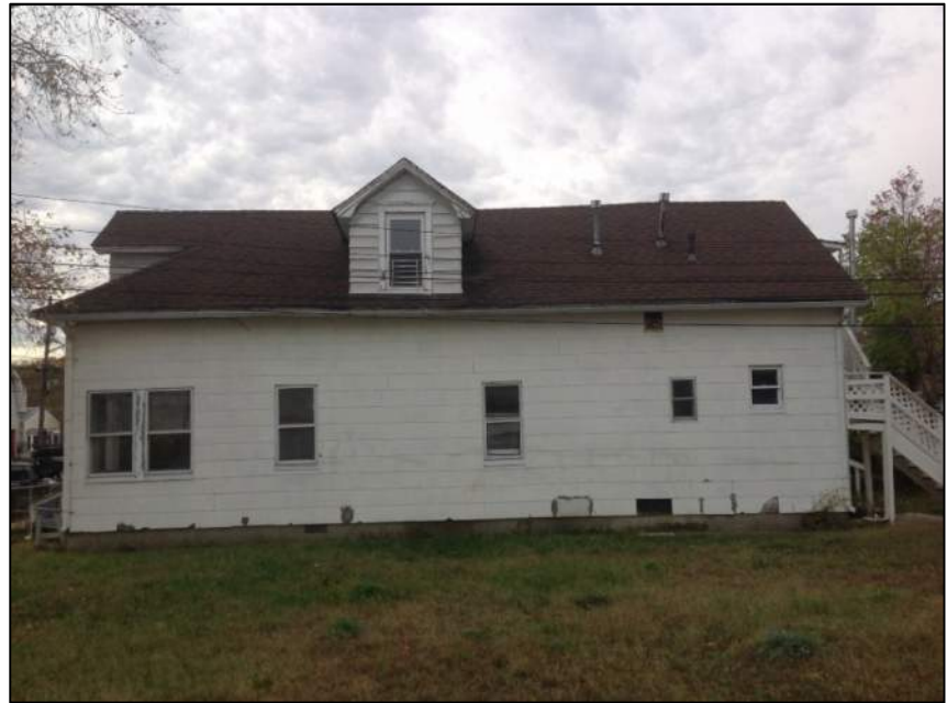
Photo 6: Right View – Building No.1
