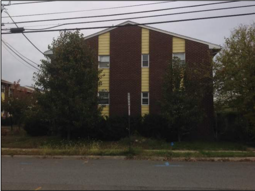
Photo 7: Front View – Building No.2
