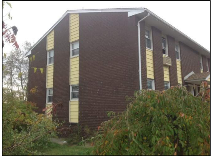
Photo 8: Rear View – Building No.2
