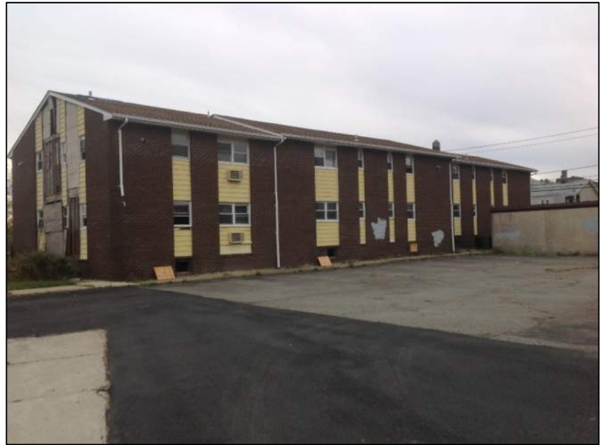
Photo 10: Right View – Building No.2
