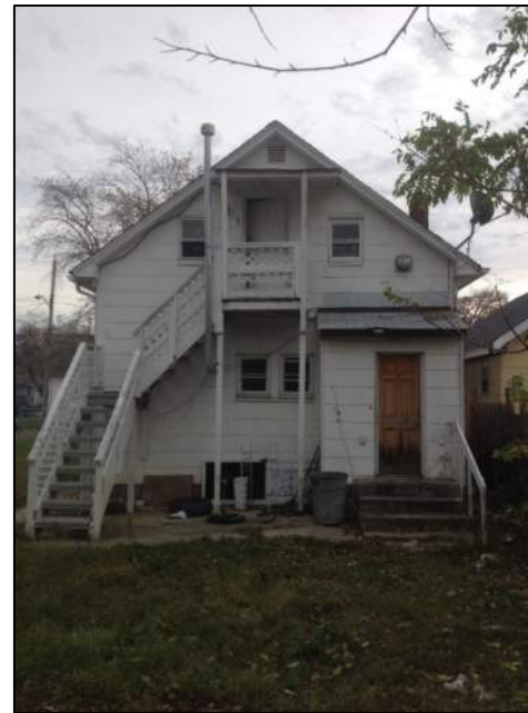
Photo 4: Rear View – Building No.1
