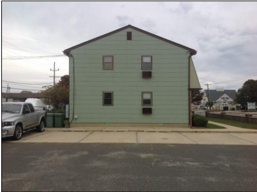
Photo 9: Left View – Building No.2
