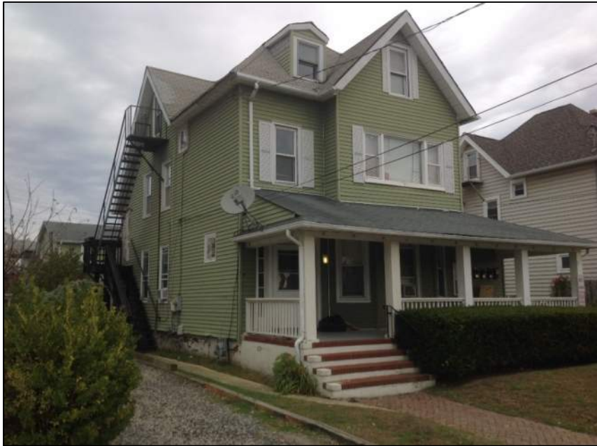
Photo 4: Left View – Building No.1
