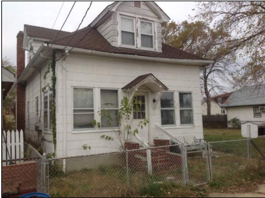
Photo 5: Left View – Building No.1
