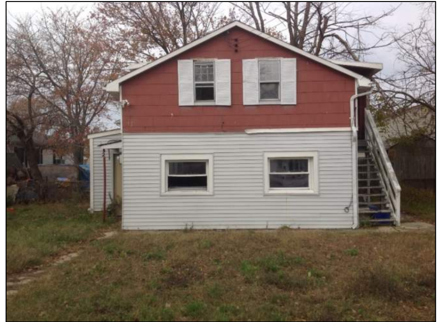
Photo 8: Front View – Building No.2
