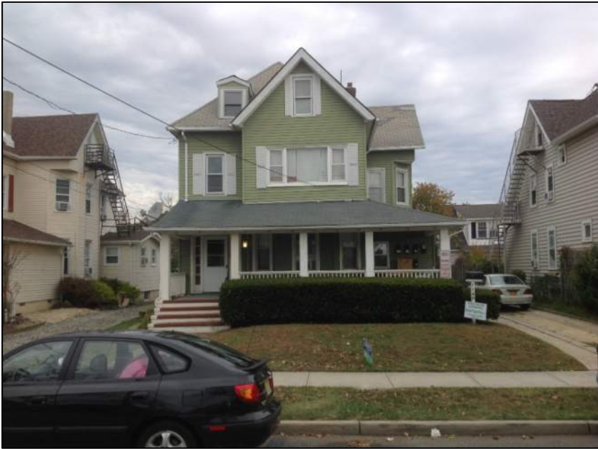
Photo 2: Front View – Building No.1
