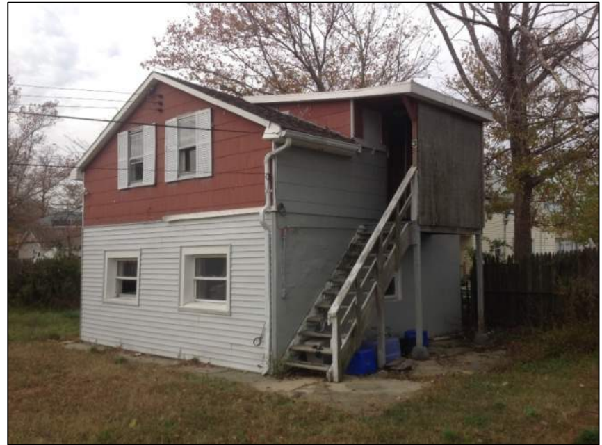
Photo 10: Right View – Building No.2
