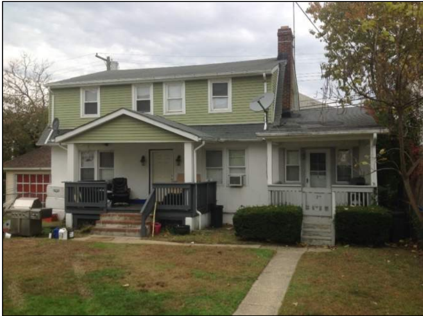
Photo 6: Front View – Building No.2
