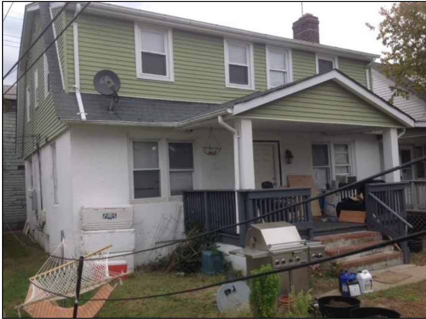
Photo 8: Left View – Building No.2
