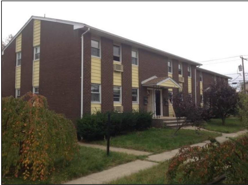
Photo 9: Left View – Building No.2
