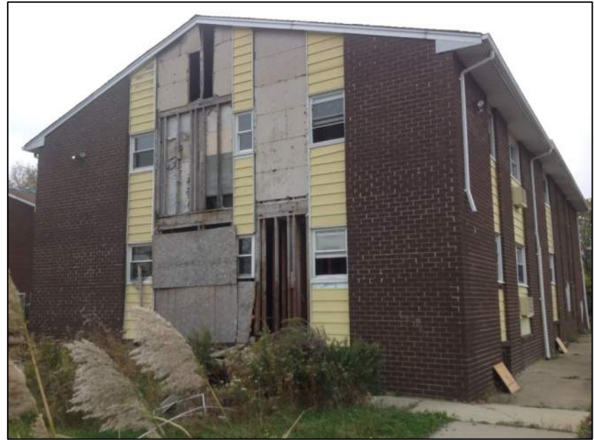
Photo 4: Rear View – Building No.1
