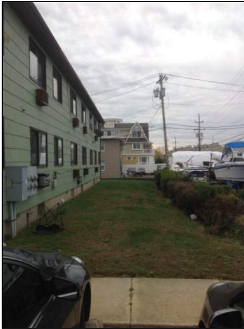
Photo 11: Backyard – Building No.1
