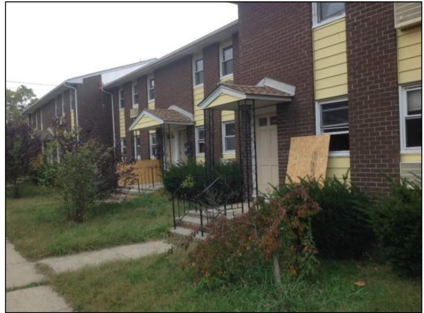
Photo 6: Right View – Building No.1
