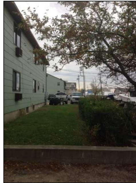
Photo 12: Backyard – Building No.2
