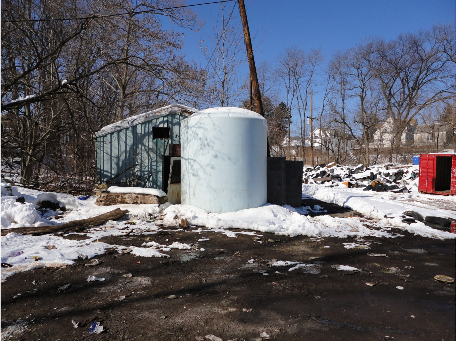
Calcium Chloride Tank
