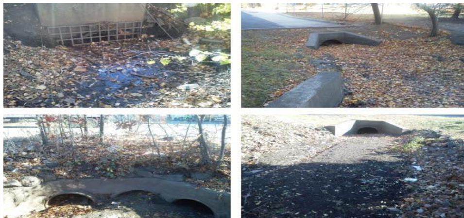
Figure 3-2: Drainage Systems, Moonachie/Little Ferry. Addressing drainage issues could offer low-cost investment opportunities to increase New Jersey’s flood resilience. For example, bottlenecks in drainage systems, accumulated debris, and overgrowth may collectively exacerbate the impact of flooding and storm surge on communities. In addition, some drainage systems, constructed piecemeal over the last two centuries, have never been mapped. For example, Rutgers has been evaluating how minor drainage improvements can reduce flooding in the Moonachie/Little Ferry region (pictured).
