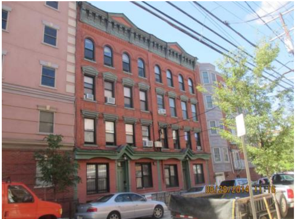
4 1 Floor Level - RRE0028738_ (31) Date Taken: 8/28/2014
