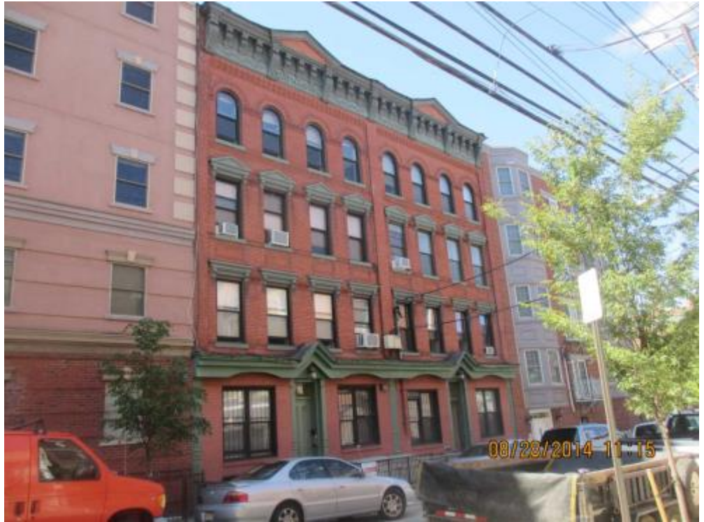
3 1 Floor Level - RRE0028738_ (30) Date Taken: 8/28/2014
