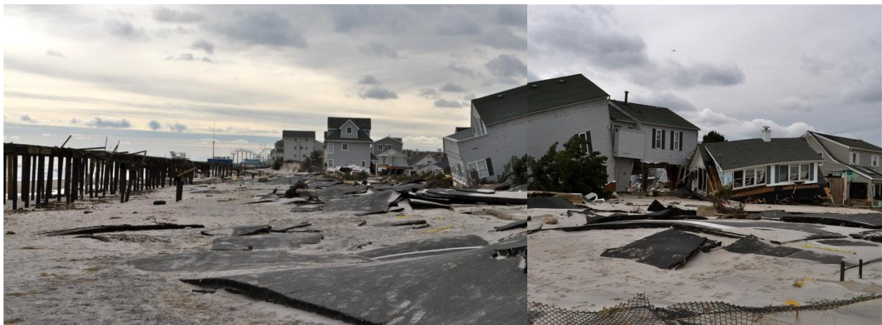
Figure 6: View of Ortley Beach boardwalk, Ocean Avenue and surrounding homes destroyed by Sandy
