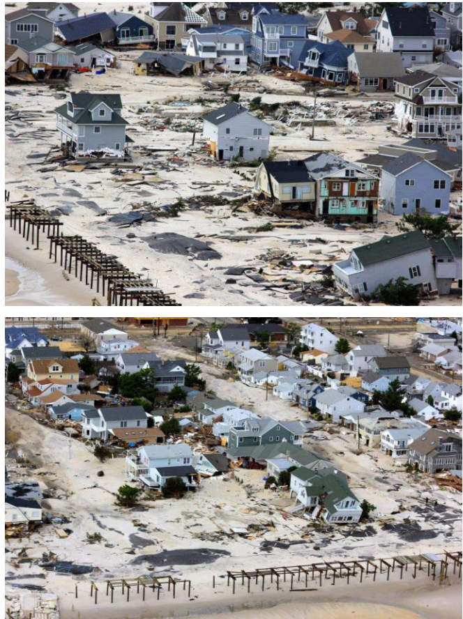
Figure 5: Aerial views of ocean side of Ortley Beach between 8th Ave and Harding Ave show many homes knocked off their foundations
