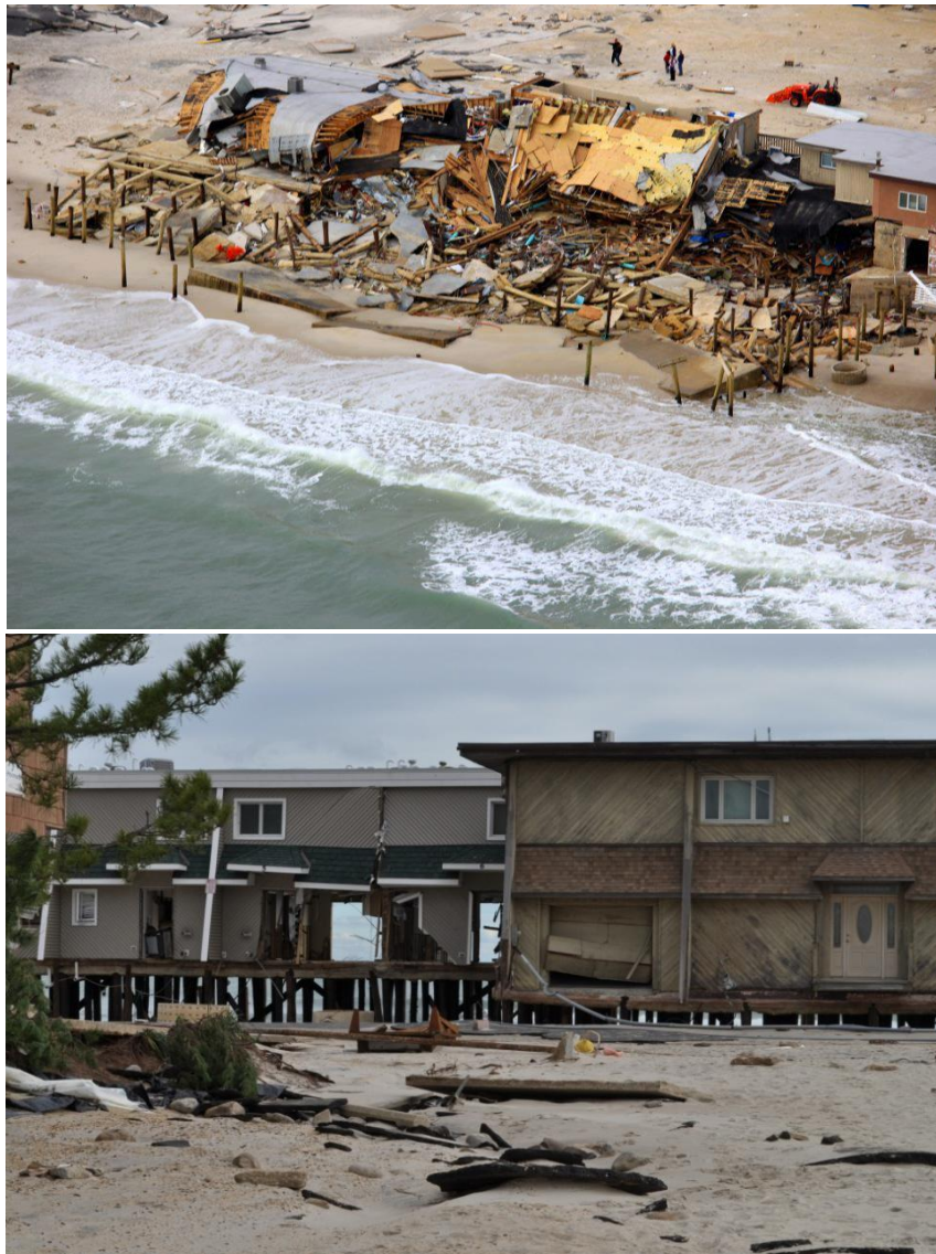
Figure 2: Images show Joey Harrison's Surf Club and Oceanside Condominiums obliterated from powerful storm surge and wave action at 6th Ave and Ocean Ave.
