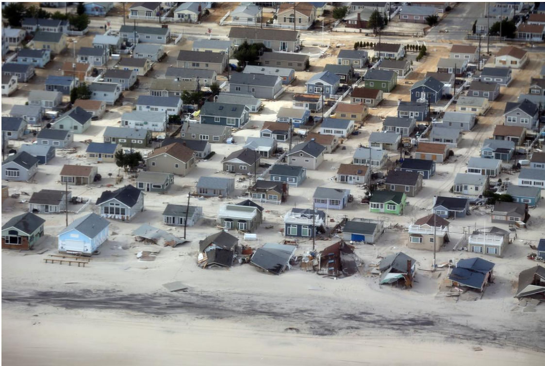
Figure 8: Ocean front properties damaged from Sandy storm surge and wave action in Dover Beaches North
