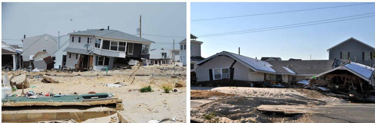
Figure 4: Ocean front properties damaged from Sandy storm surge and wave action in Ortley Beach
