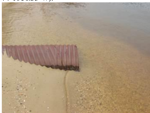
Figure 2. Storm pipe at Site 2 of Beachwood Beach West.
