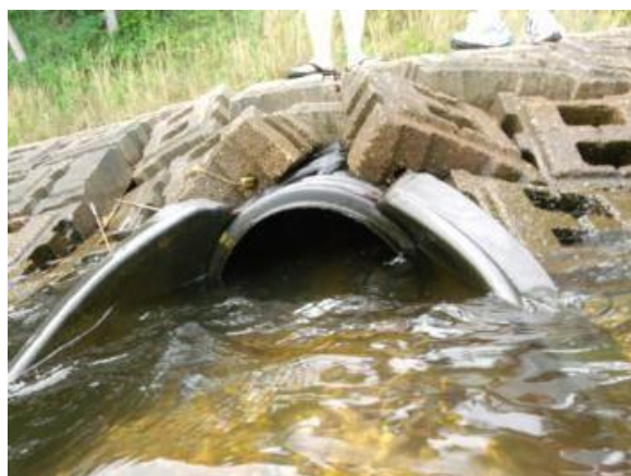
Figure 3. Storm pipe at Site 4 of Beachwood Beach West.
