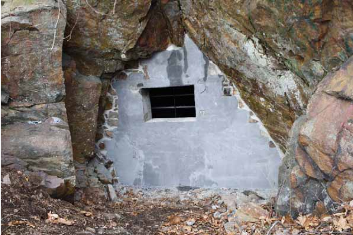
Figure 1. The completed bat conservation gate at Dolan Tunnel.
