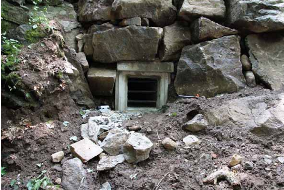
Figure 2. Retaining wall and box culvert with bat conservation gate at Hibernia Mine.
