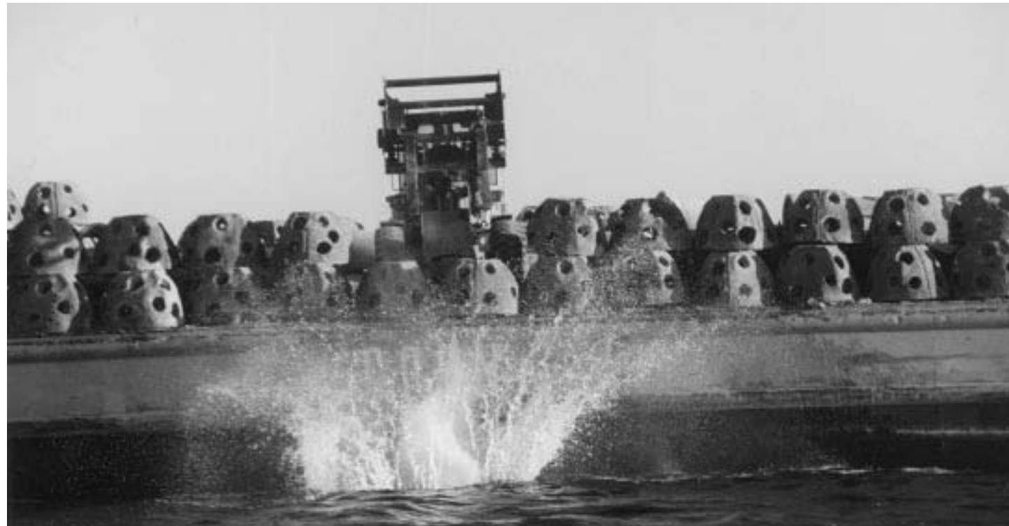
While hundreds of Reef Balls were placed on the Cape May and Wildwood Reef Sites, each one is important, since each Reef Ball functions individually as a micro-reef, fostering its own population of fish and marine life.
