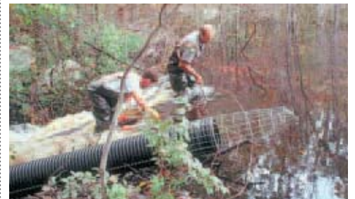
Fish and Wildlife technicians installing a "flume" at Silver Lake Wildlife Management Area.
