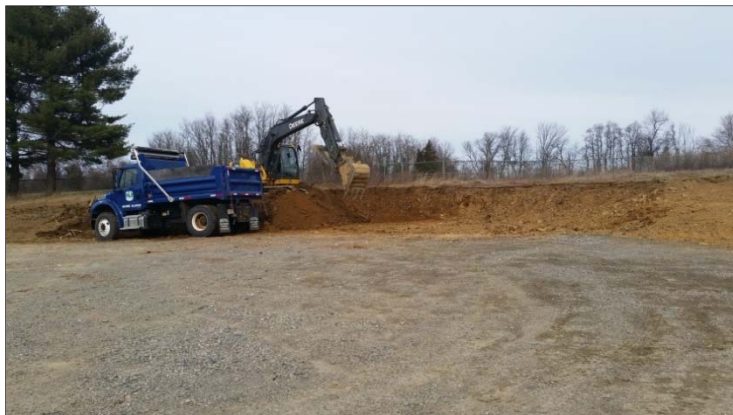
Creating a slope for erosion control at the RVR boat ramp site.
