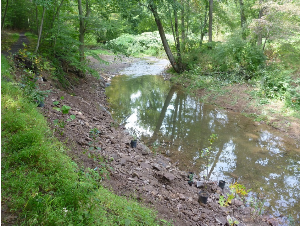
Restored bank, looking upstream, showing native trees ready to be planted and new pool.
