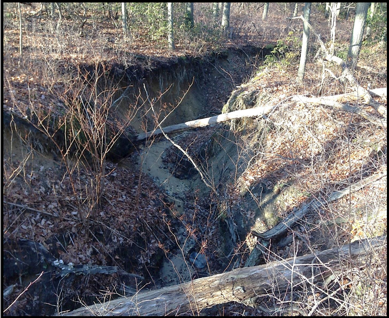
Figure 14.3: Surface Erosional Channel Resulting from an Improperly Designed Stormwater Pipe
