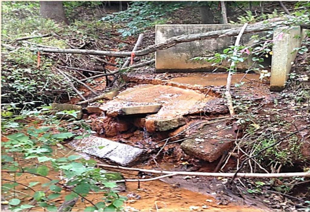
Figure 14.2: Erosion Due to Insufficient Pipe Pitch
