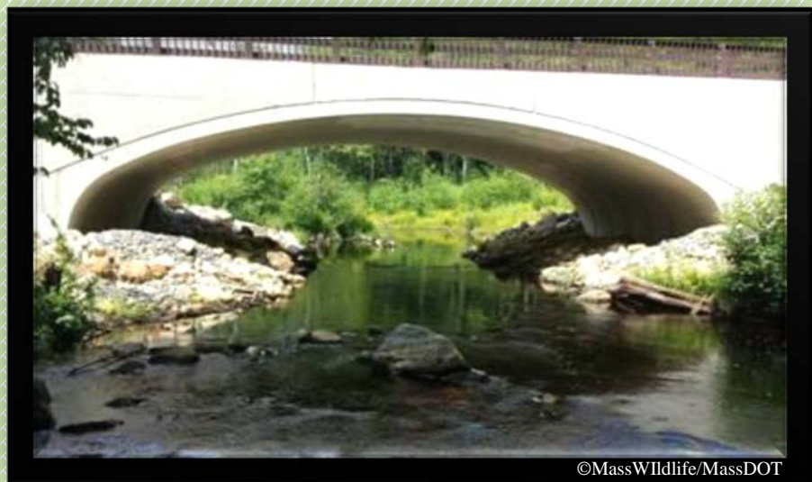
Figure 10.19: Bridge Replacement at 1.2 Times Bankfull Width for Installation of Wildlife Passage
