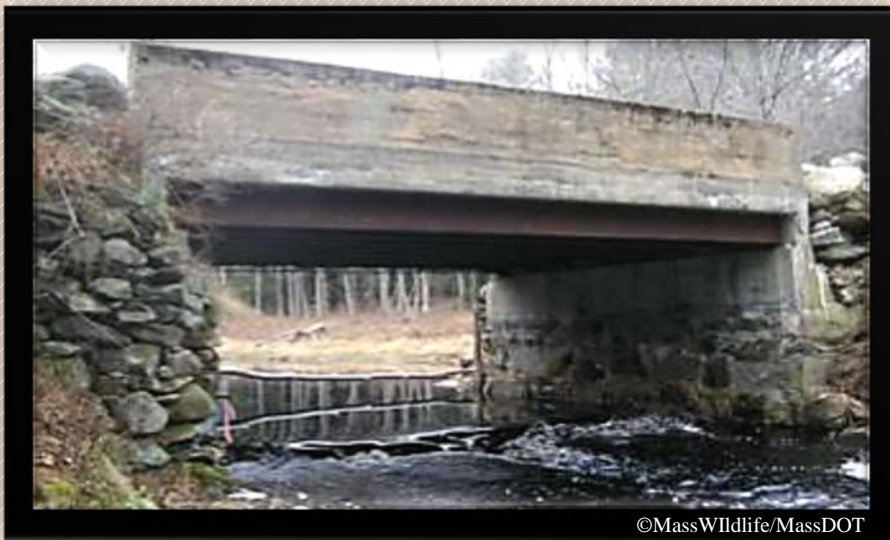
Figure 10.18: Bridge Before Installation of Wildlife Passage
