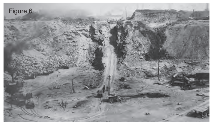
Figure 4, 5 and 6. Quarry and works of the Alpha Portland Cement Company, from Annual Report of the State Geologist for the Year 1903. Figure 4 shows the cement plant and figures 5 and 6 show the quarry. Photos from NJGWS archives.
