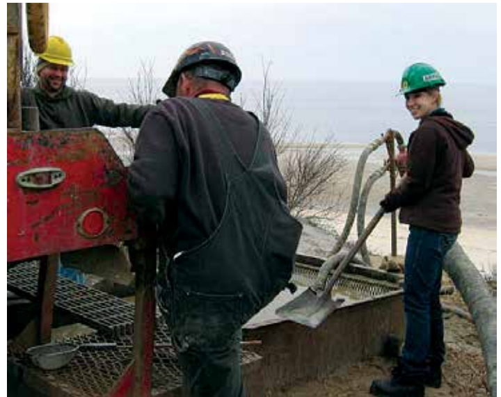
Figure 4. Drillers constructing an observation well along Cape May's Delaware Bay shoreline. Photo by S.W. Johnson
