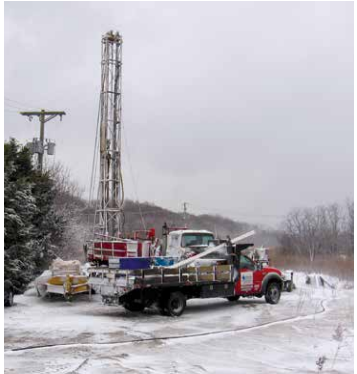
Well driller uses a mud-rotary drilling rig to construct a 250-foot deep sentinel observation well in the Cohansey aquifer beneath Cape May County. Photo by S.W. Johnson
