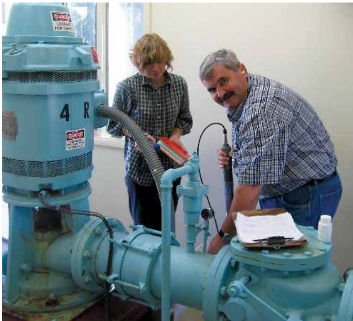
Figure 7. Yelena Stroiteleva, Hydrogeologist, and Ovidiu Petriman, Principal Geologist, collect and field analyze groundwater samples from Atlantic City 800-foot sand aquifer water-supply well. Photo by S.W. Johnson
