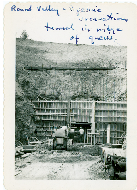
Figure 5. Pipeline excavation tunnel in ridge of gneiss, date unknown, photographer unknown .
