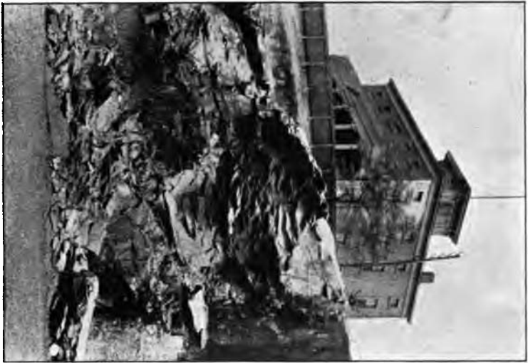
Fig. 1. Concentric jointing in diabase. Pa. R. R. cut, Jersey City. (Orphans' Home, beyond, is built of diabase.)
