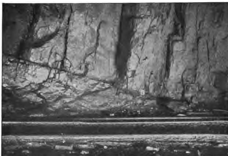
Fig. 2. Lower contact of Palisade diabase on sandstone (arkose), Pa. R. R. tunnels, Weehawken, 50 feet below mean high tide. The diabase exhibits the typical rectangular jointing. (Reproduced by courtesy of Chas. M. Jacobs, Chief Engineer.)
