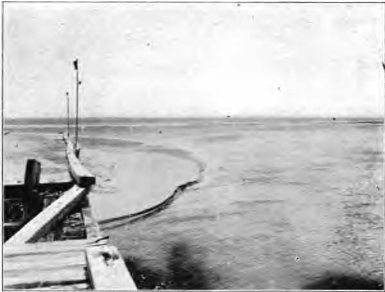
Fig. 1. Outer end of north dike in July, when it was surrounded by a sand bar extending 150 feet seaward of its outer end.
