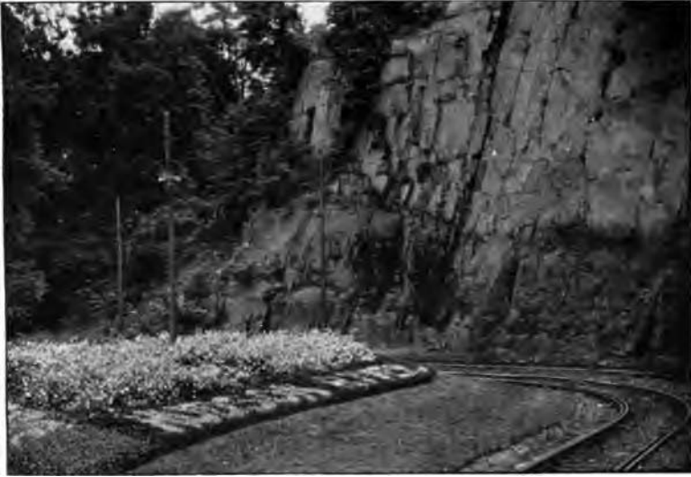
Fig. 1. Olivine-diabase ledge in railway cut back of Fort Lee. The normal diabase above shows typical rectangular jointing.
