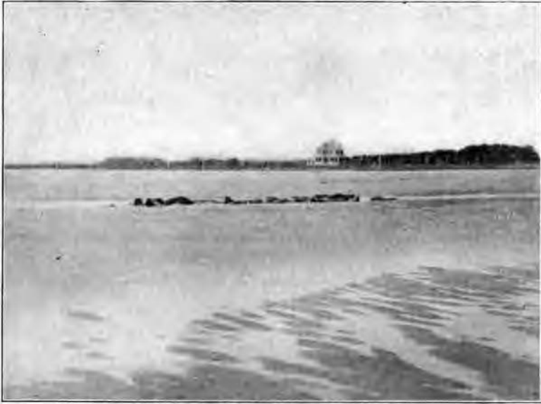
Fig. 1. Remains of south dike at low water in Manasquan entrance, looking southwest from the north dike.
