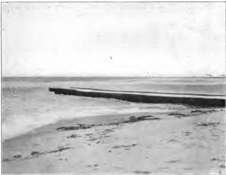
Fig. 2. Is a view taken August 28th, from a point on the beach north of the Manasquan, Government dike, looking southeast, across the inlet and the outer end of the sand-spit on the Point Pleasant side, and showing the erosion at the outer end of the dike, due to a northeast storm.
