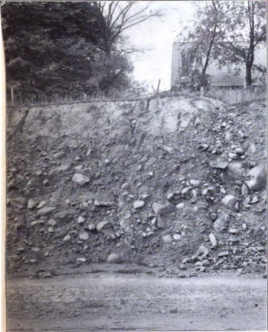
Section showing the physical heterogeneity of the drift in the northeast part of Newark.
