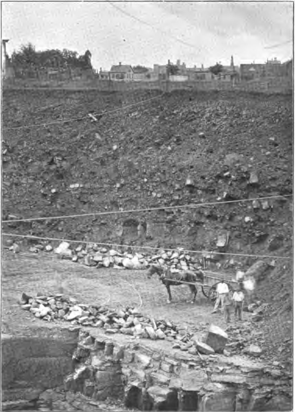
Till over sandstone. Quarry in Newark. The till is made up largely of local, angular stones.
