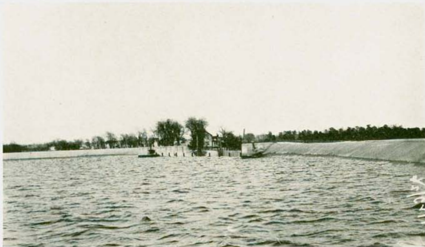
Absecon Pond, source of part of public water supply for Atlantic City.
