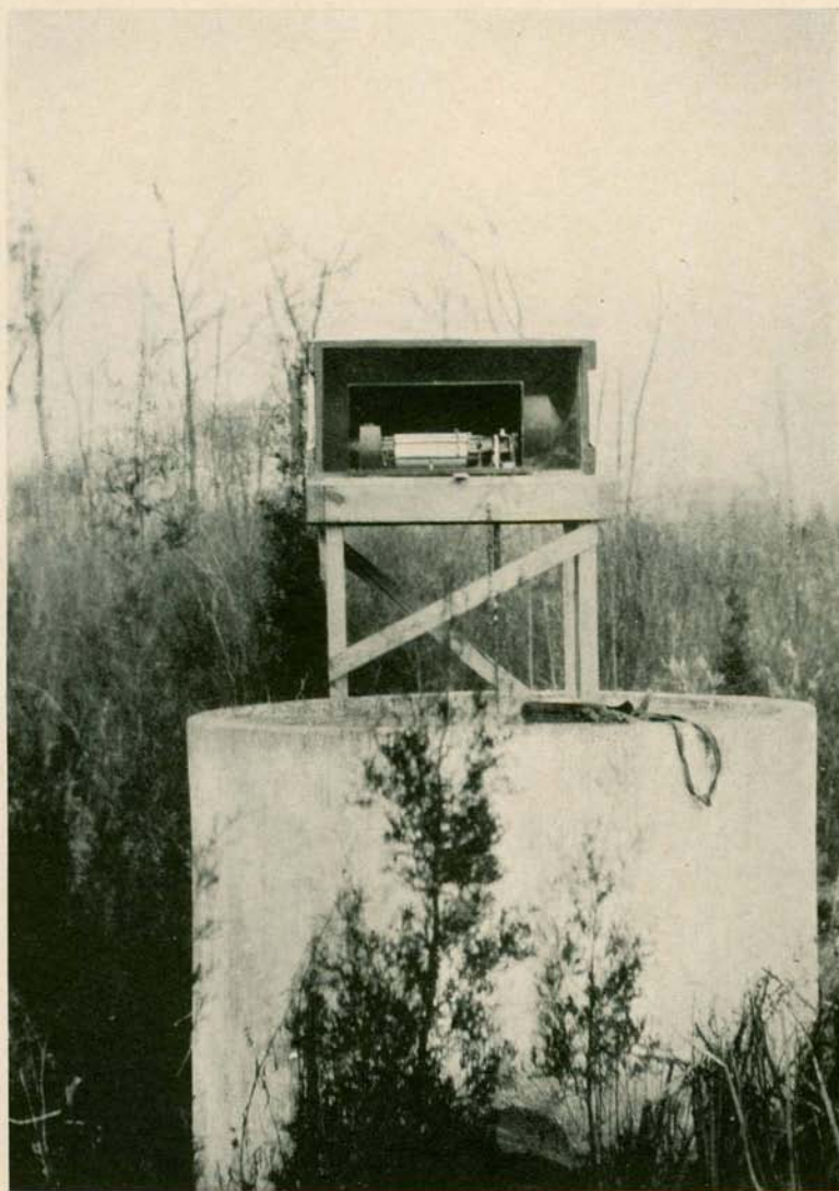
Water-level recorder installation on well No. 28, Atlantic City Water Works well field.
