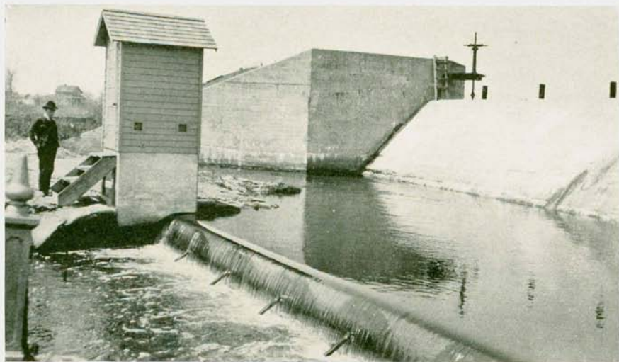
Weir and gaging station below Absecon dam, maintained by New Jersey Department of Conservation and Development and U. S. Geological Survey to measure flow of Absecon Creek.
