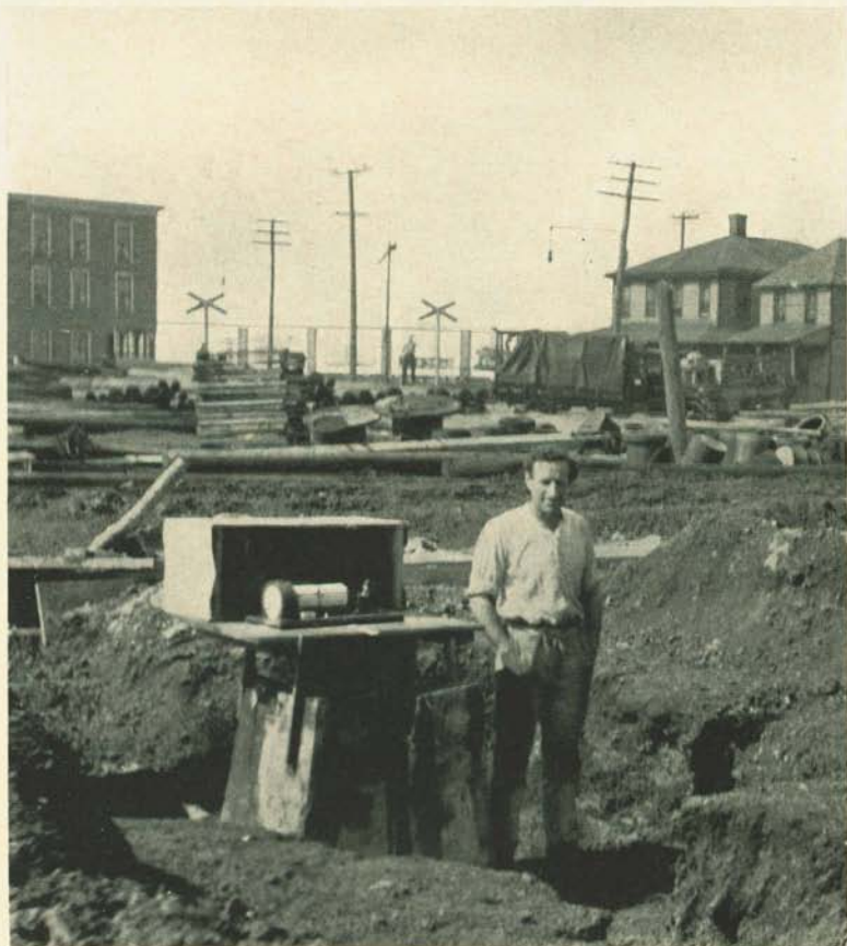
Temporary installation of water-level recorder on new well of Atlantic City Electric Co., May, 1924.
