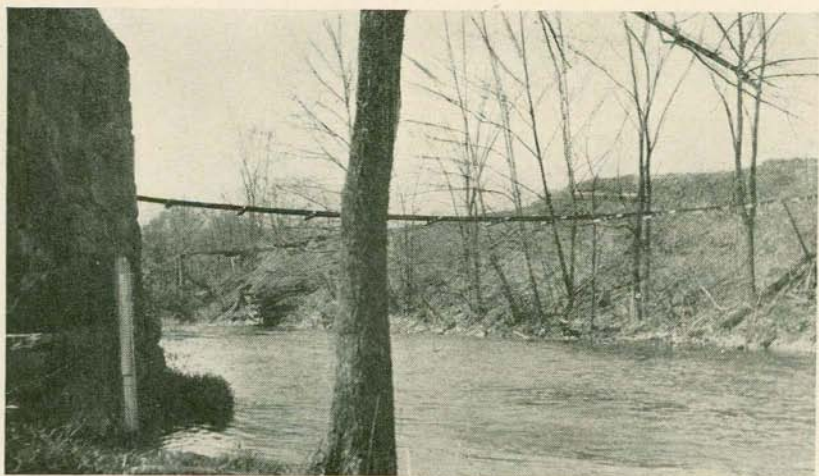
(b) Gaging bridge.
