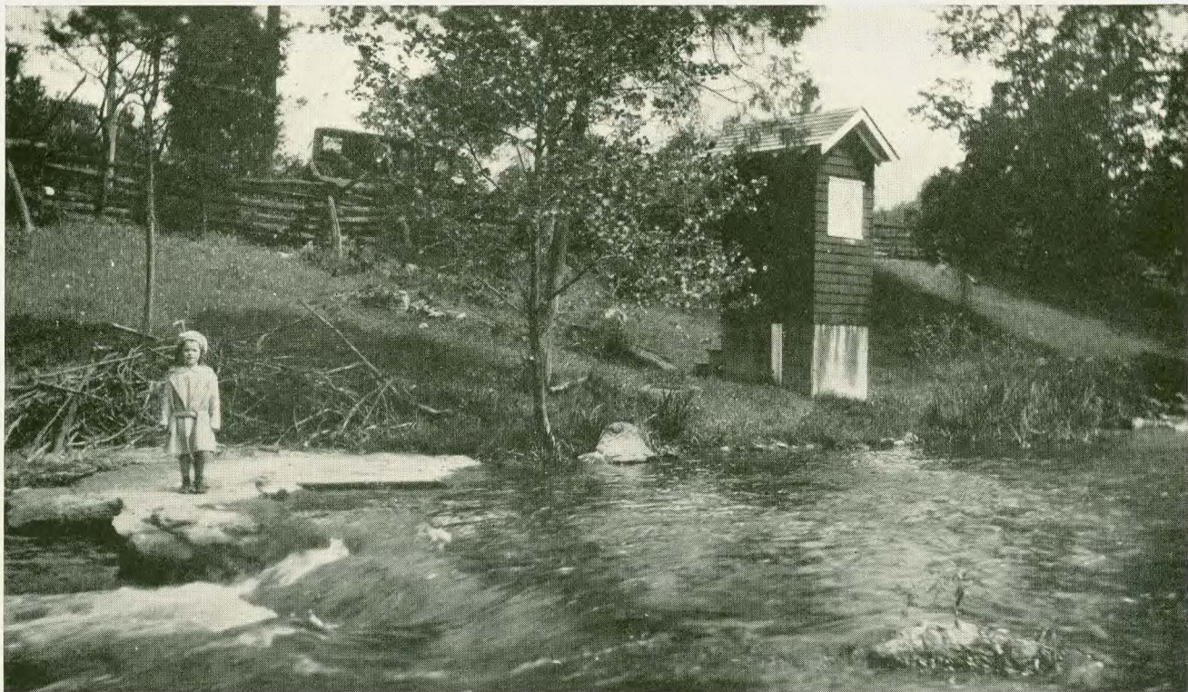
Gaging station on Beaver Brook near Belvidere, shelter for automatic water-stage recorder, natural control shown in foreground.
