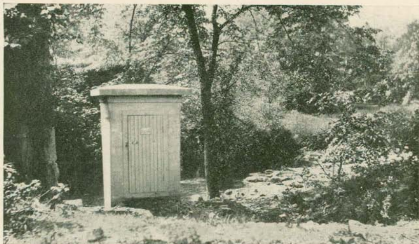
(a) Shelter for automatic water-stage recorder.
