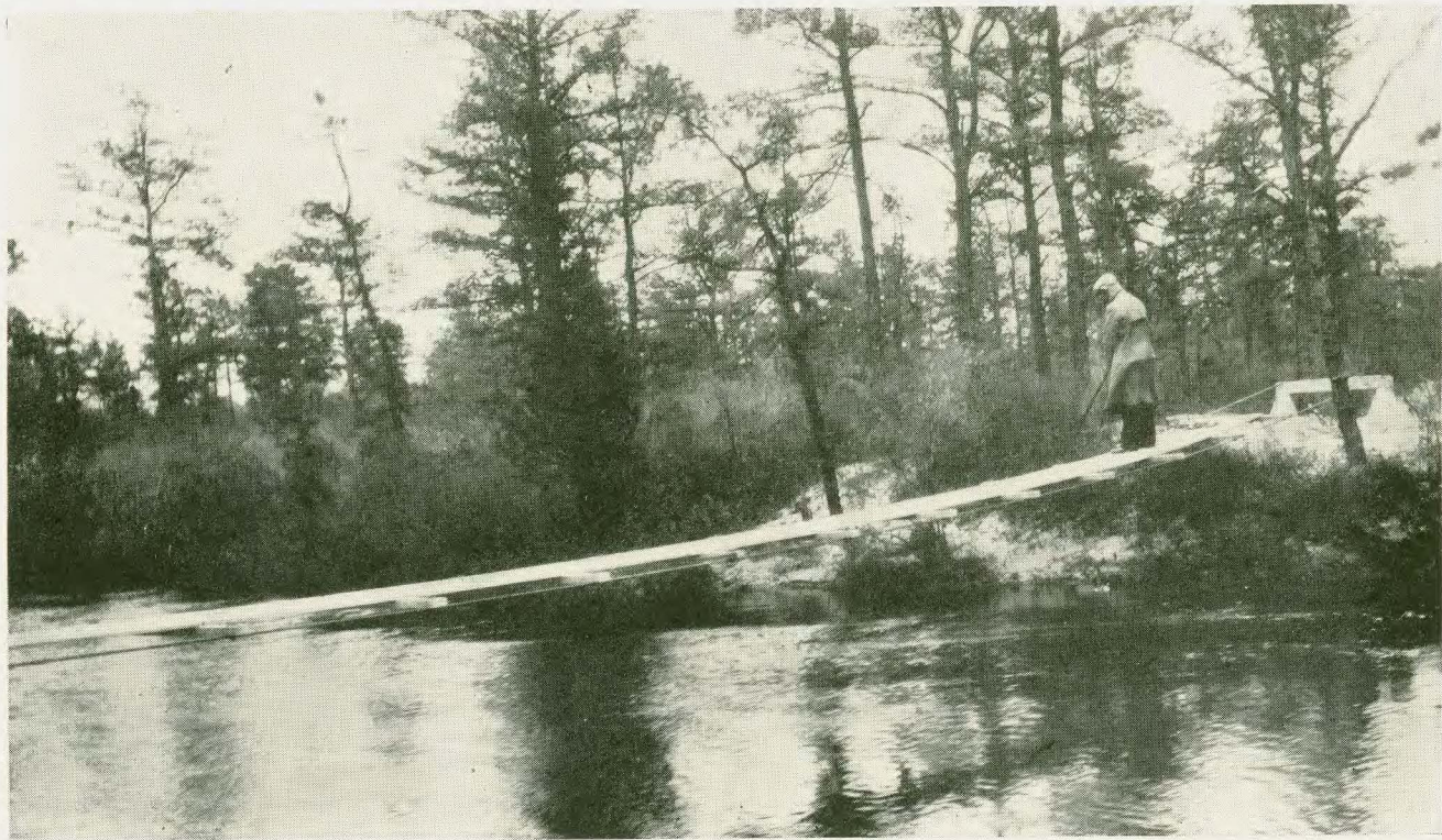
Engineer making flow measurement from gaging bridge. NEW JERSEY GEOLOGICAL SURVEY
