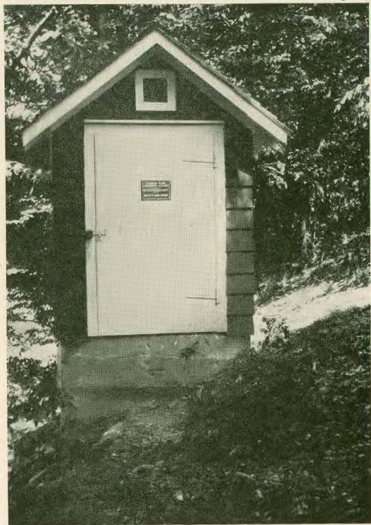
(a) Shelter for automatic water-stage recorder.
